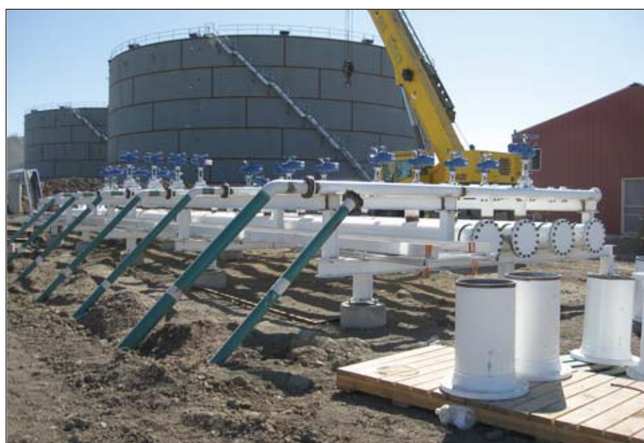
The tank and receipt and delivery manifold for all truck and pipeline movements in and out of the COLT Hub. Three of the five crude oil storage tanks are visible in the background.
