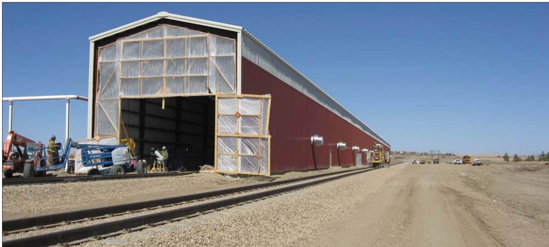
Exterior view of the rail loading canopy at COLT. Loading will initially be done through 10 loading arms. Plans are underway to add four additional loading arms.
