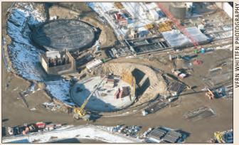
Construction continued in December on the first phase of a new wastewater treatment facility for Williston, North Dakota. The first phase, expected to be competed in September, will have capacity for a population of 40,000, and components have been installed to up the capacity for a population of 60,000. The site has expansion potential for a population of 120,000.
