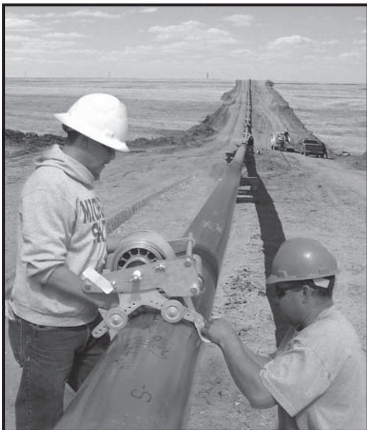
One of thousands of projects using Polyguard RD-6 non-shielding coating. Our first was in 1988.
