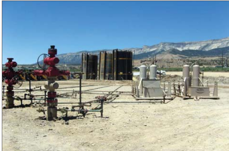
From a Colorado Oil and Gas Conservation Commission brochure, pictured above is green completion equipment in an unidentified field in Colorado.
