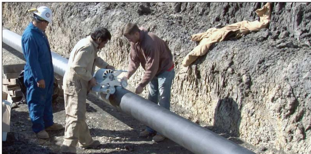
Polyguard RD-6 applied during a rehabilitation job.
