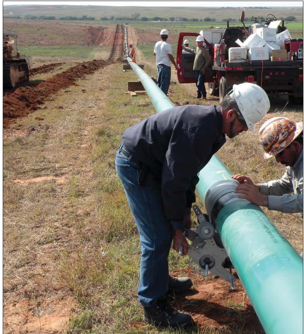
Girth weld application of Polyguard RD-6 on a miles and miles of pipe.
