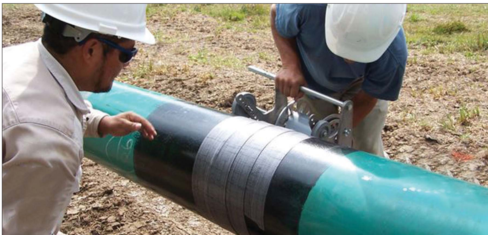
Installation of Polyguard RD-6 on a girth weld.
