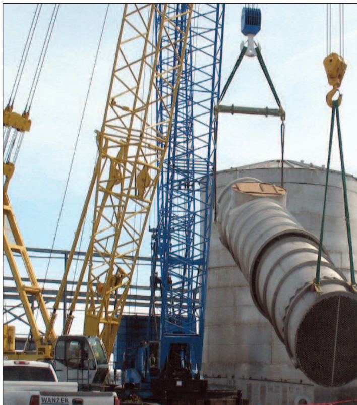
Whether new construction, regular maintenance, planned outages or emergencies, Wanzek is responding to the increasing demand for electricity in North Dakota and throughout the U.S.
