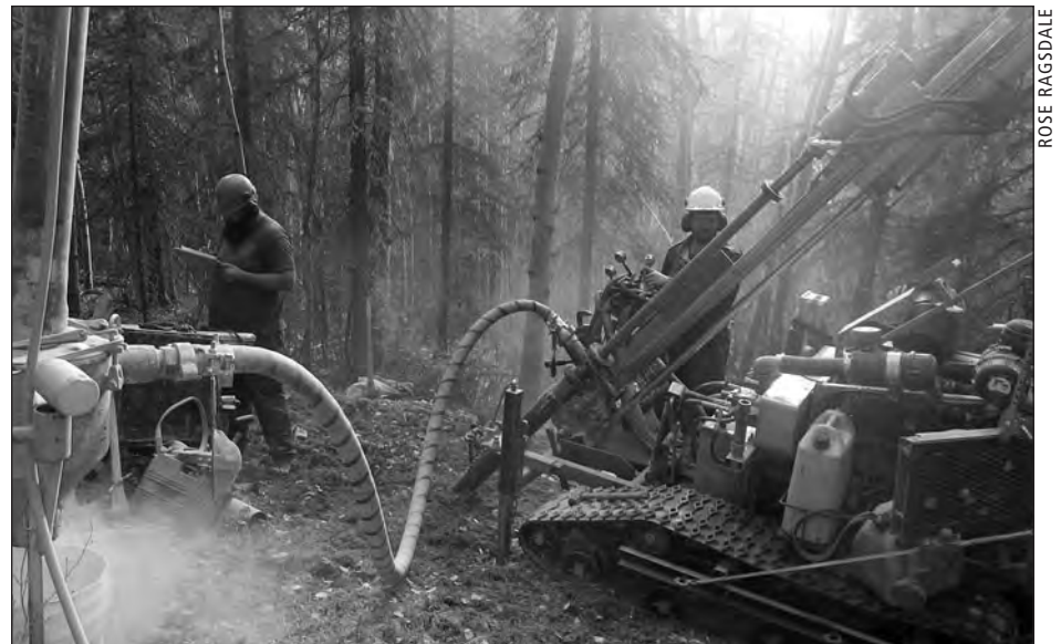
The RAB (rotary air blast drill) is a third component in the package of services that Groundtruth Exploration Ltd. has designed for early-stage mineral exploration. The relatively lightweight drill can obtain bedrock core samples down to nine meters.
