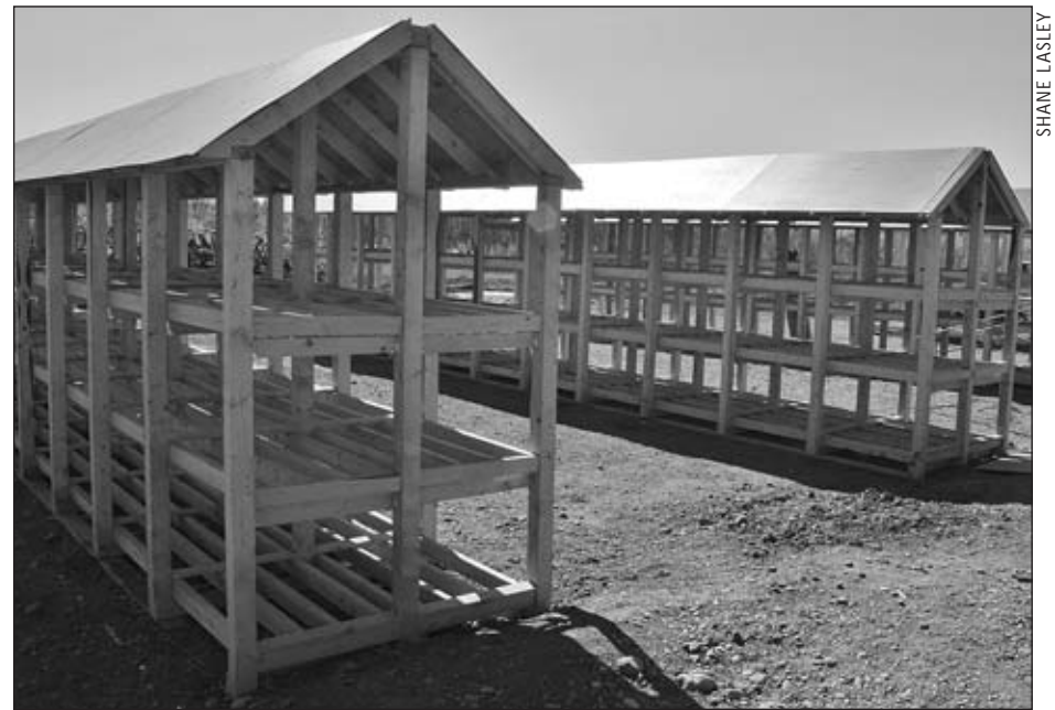
These newly built core shacks were constructed in anticipation of the more than 47,000 feet (14,000 meters) of drilling completed at the Tetlin gold-copper-silver project during 2013.
