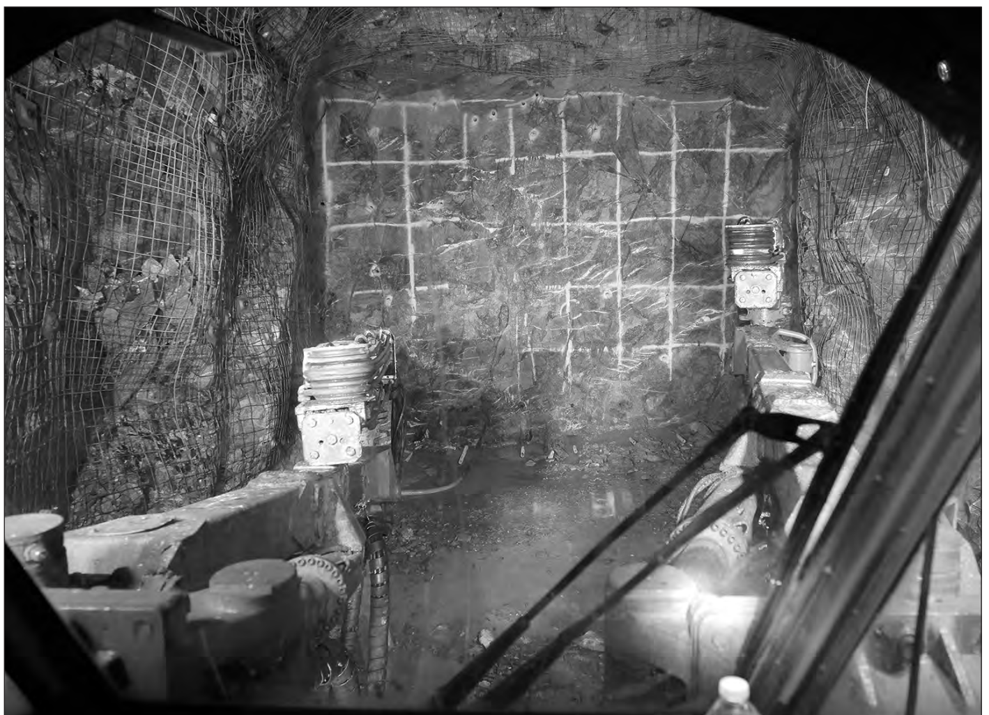
Underground development reached the Jualin deposit at Kensington during the third quarter and this higher grade ore is expected to help boost gold production at the Southeast Alaska operation moving forward.
