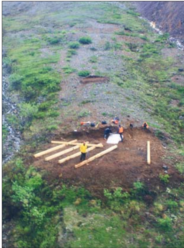
This pad being constructed in late June at the Grubstake prospect is the site of the first hole drilled this year at Corvus Gold Corp.'s Chisna porphyry copper-gold project.
