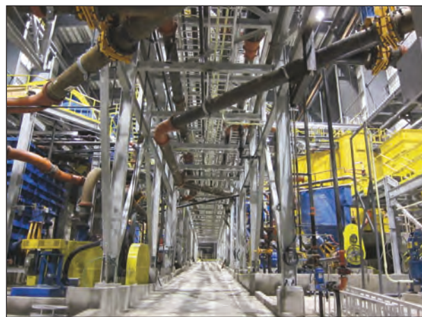
The flotation bay at Imperial Metals’ Red Chris Mine was ready for commissioning at the time of this October photo. The northwestern B.C. mine plugged into the power grid in November and the electrical components are being tested in anticipation of a December startup.
