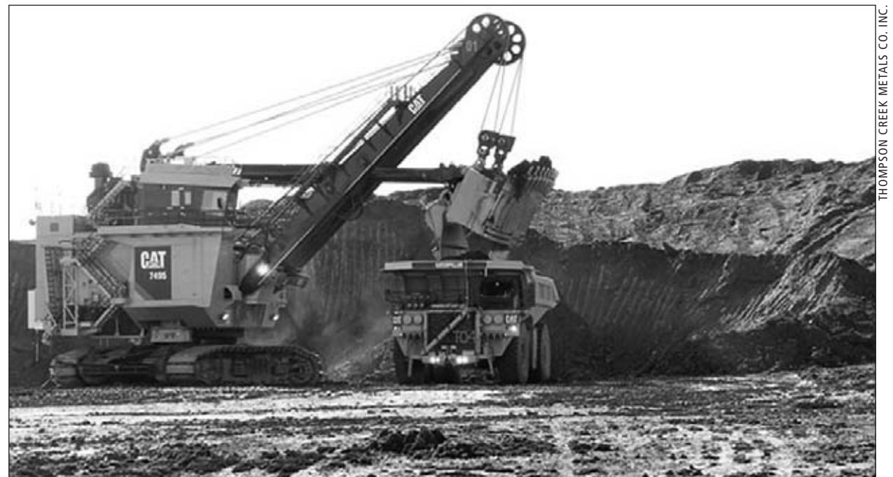
The Mount Milligan copper-gold mine project in north-central British Columbia is scheduled to begin production in August with a 60,000-metric-tons-per-day open pit operation with a 22-year mine life. The project's mine pit and mobile equipment, including two electric shovels and a fleet of trucks, is already fully operational.
