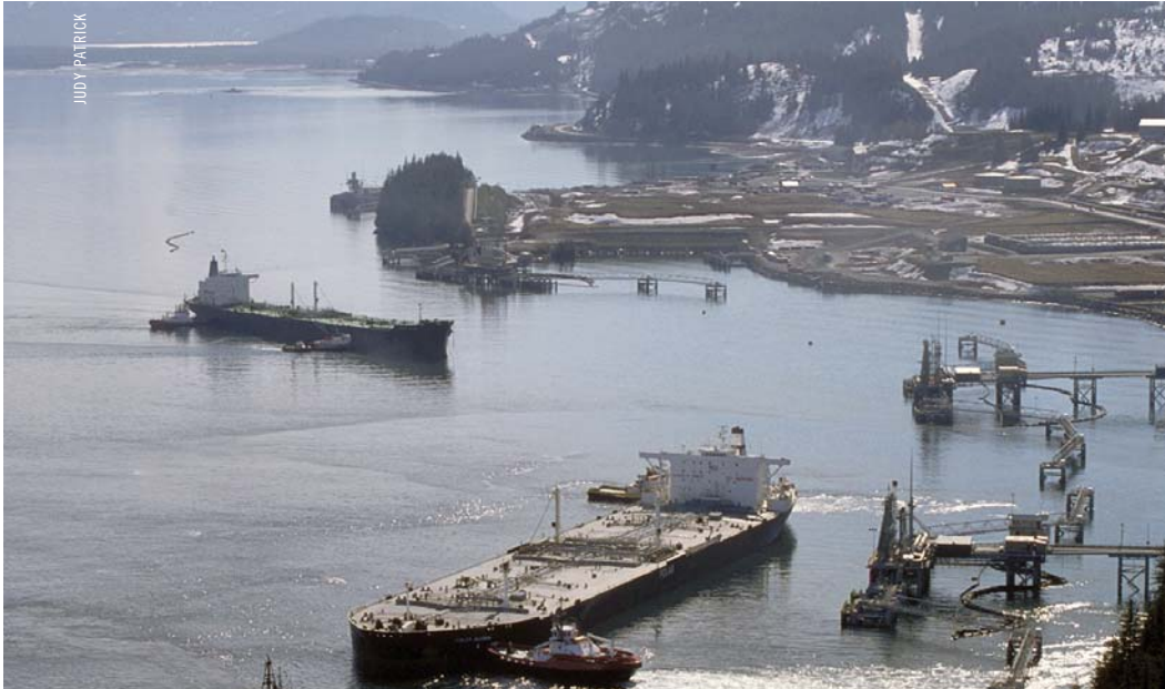
Oil tanker receiving terminal at Port of Valdez in Southcentral Alaska. The 800-mile trans-Alaska oil pipeline starts at Prudhoe Bay on the North Slope and terminates here.
