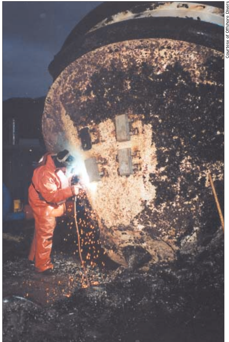
Offshore Divers welders replacing anodes on a mooring buoy (15-feet in diameter) for spill response in Valdez.
