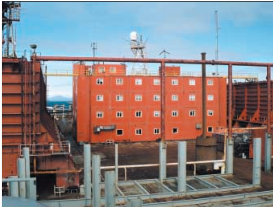
According to Fairweather Inc., the drilling mast and substructure has "a rated capacity of 1.3 million pounds and can readily be skidded to drill through any one of the four moon pools." The SDC has 6 Caterpillar D399, 1,000 horsepower engines.
