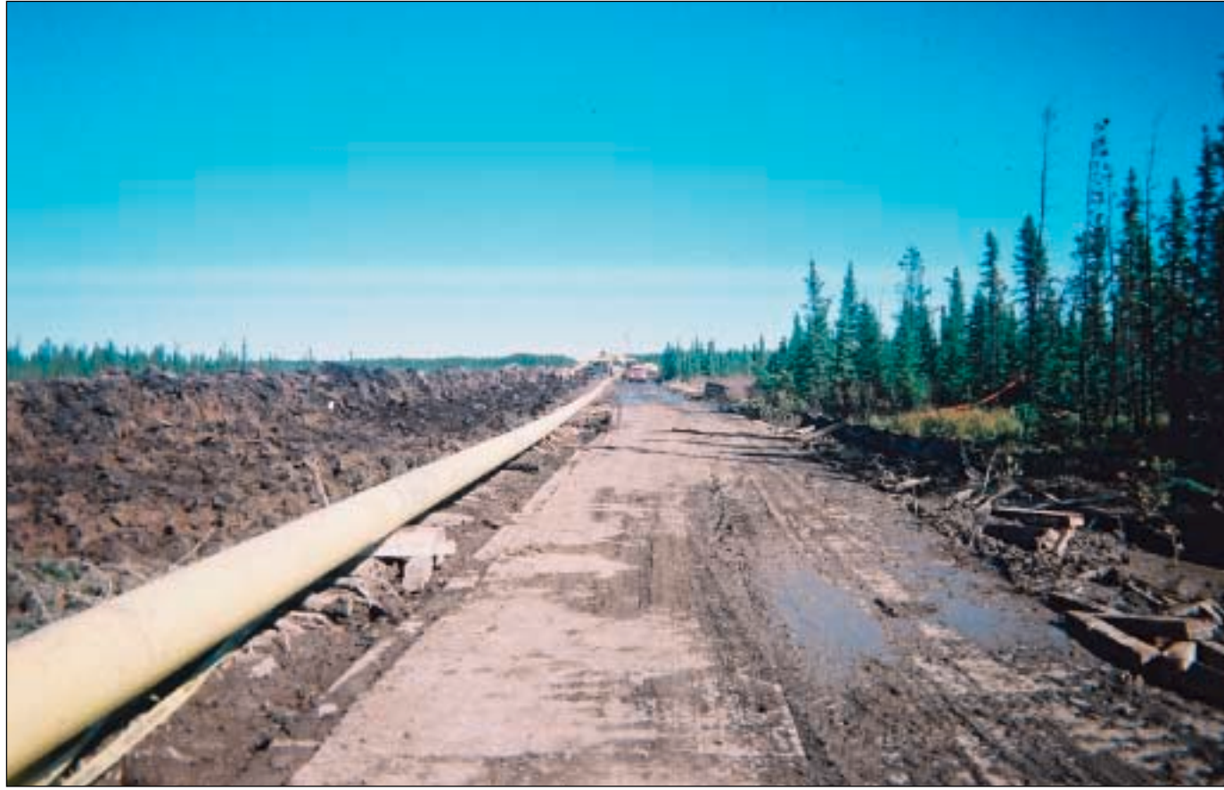
Mats minimize the impact to the natural landscape with DURA-BASE utilization. The mats measure 8 feet by 14 feet and are designed with overlapping lips that combine with a drop-in locking pin to bind the entire mat system together into a solid surface for roads, operational pads and staging areas on soft sub-grades.
