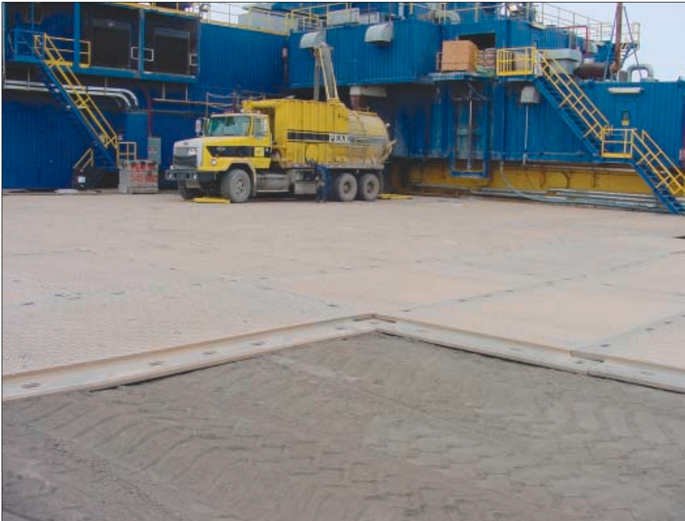
DURA-BASE onsite in Prudhoe Bay. DURA-BASE is a proprietary product substituting systems currently utilized as site-preparation methods in the Arctic environment.
