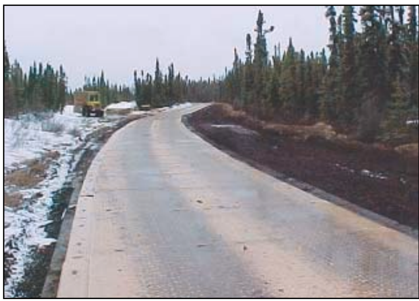
DURA-BASE provides all-weather, all-season access roads.
