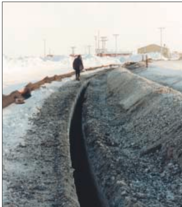
During the 1995 replacement of the four-inch main gas distribution line, Conam workers laid 6.5 miles of polyethylene coated six-inch steel mainline pipe combined with a variety of four and two inch subheader and lateral lines.
