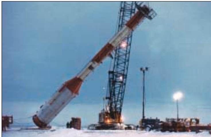
Replacement of the flare stack at pump station number one in Prudhoe Bay in 1986 was completed in two phases. In the second phase, the new flare stack was lifted into place as a single completed section. The project was completed 28 days ahead of its contractual requirements.
