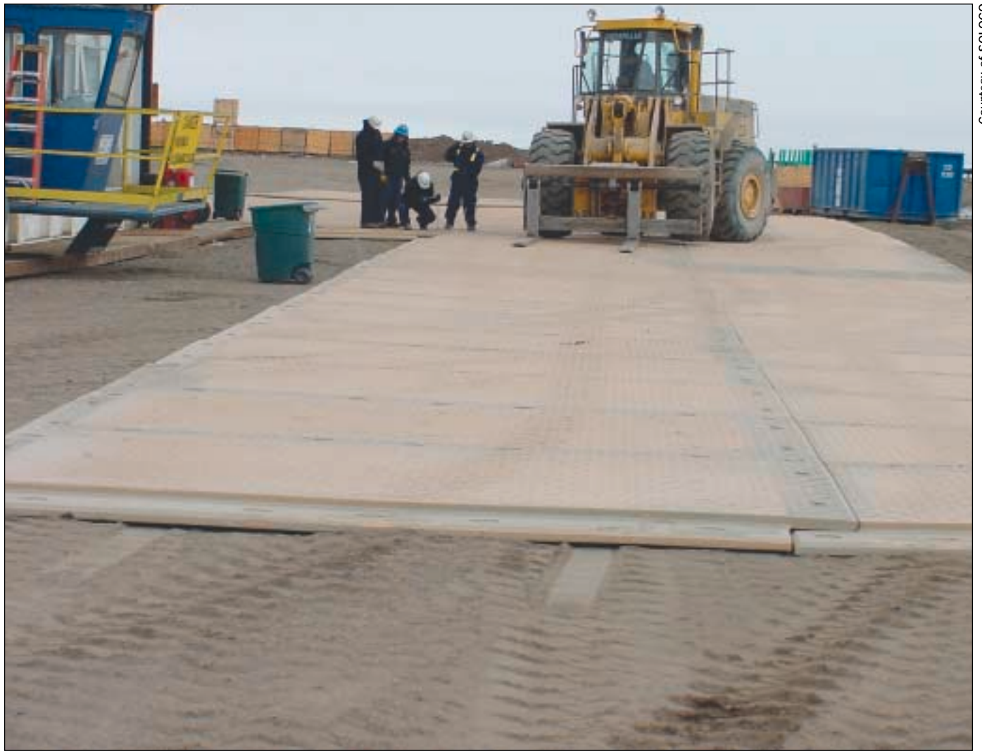
Mats minimize the impact to the natural landscape with DURA-BASE utilization. The mats measure 8 feet by 14 feet and are designed with overlapping lips that combine with a drop-in locking pin to bind the entire mat system together into a solid surface for roads, operational pads and staging areas on soft sub-grades.
