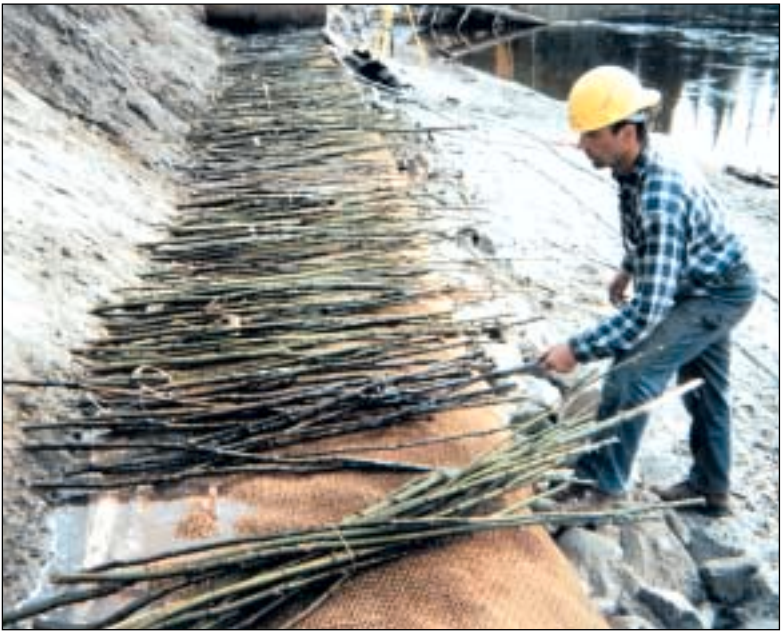
At left, Great Northwest employees use state-of-the-art construction equipment while on the job. Asphalt is being laid out by one of the 400 pieces of machinery in the company's $10 million fleet. Above, workers control erosion along the Chena River by placing small rock rip rap, burlap and willow tree cuttings.
