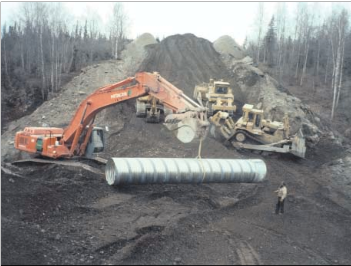
A 12-foot diameter culvert is replaced as part of the Dalton Highway milepost 144 to 175 reconstruction project. More than a million cubic yards of gravel were mined, hauled and placed as part of this project.
