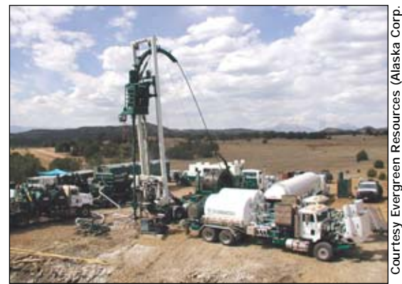
Pictured here is Evergreen's coiled tubing unit used for well completions.
