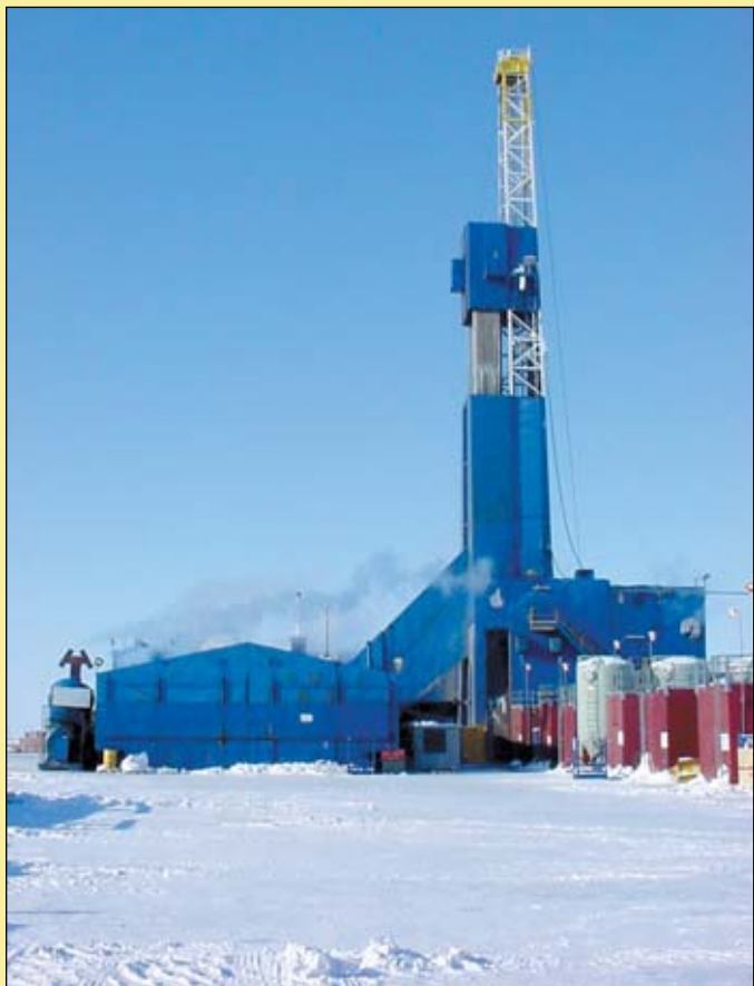
Courtesy Nabors Alaska Drilling
