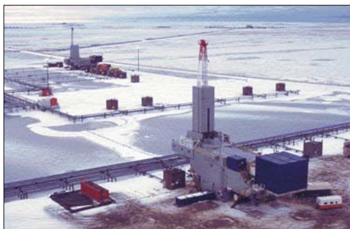
Schlumberger's Nordic 2 rig. Drilling with coiled tubing is now used for nearly half of all new wells on the North Slope. Wells can be sidetracked at lower cost than with conventional drilling rigs.
