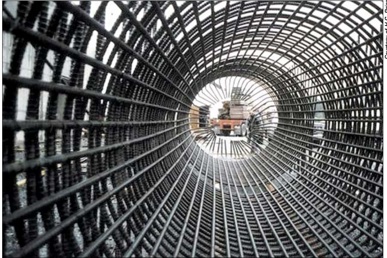
Site assembled, reinforced steel for the Healy Clean Coal Project.
