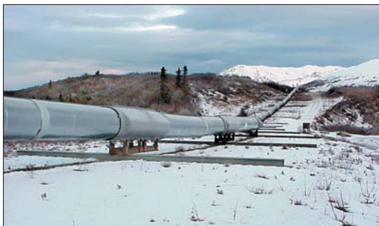
The trans Alaska pipeline, showing the special supports to accommodate movement on the Denali fault.
