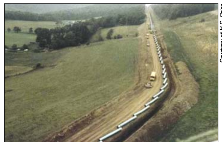
Stringing pipe on a large diameter pipeline in northern Canada.
