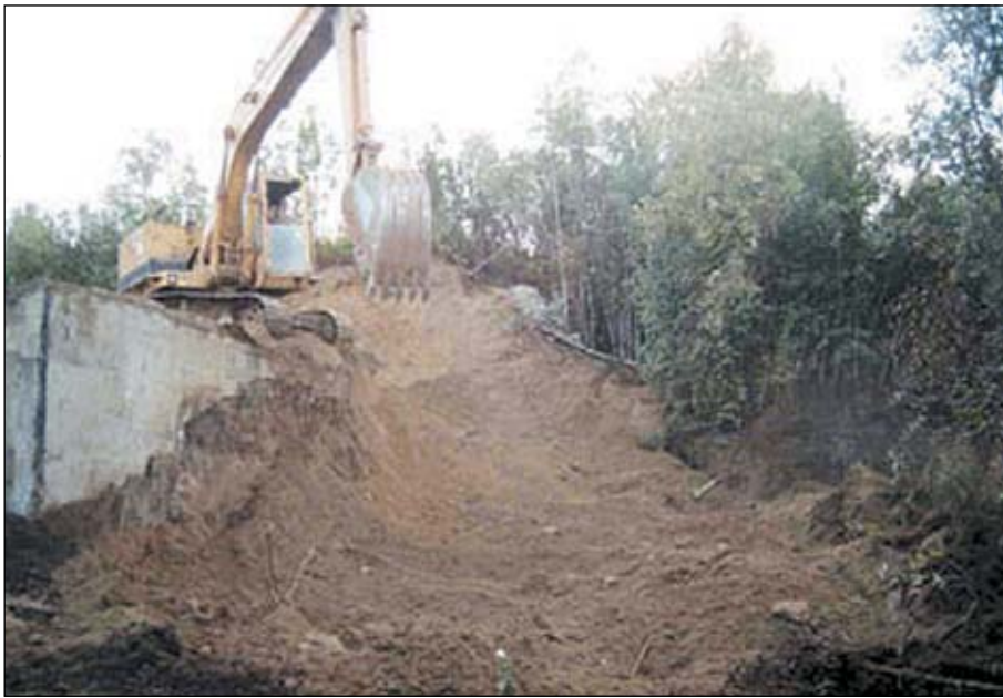
Pictured is the Four Bears Site where the buried railroad tank car was removed and the diesel contaminated soil caused by the leak in the tanker car was located. This backhoe is removing the contaminated soil, loading it into a truck that is bring the soil to the on-site remediation location.
