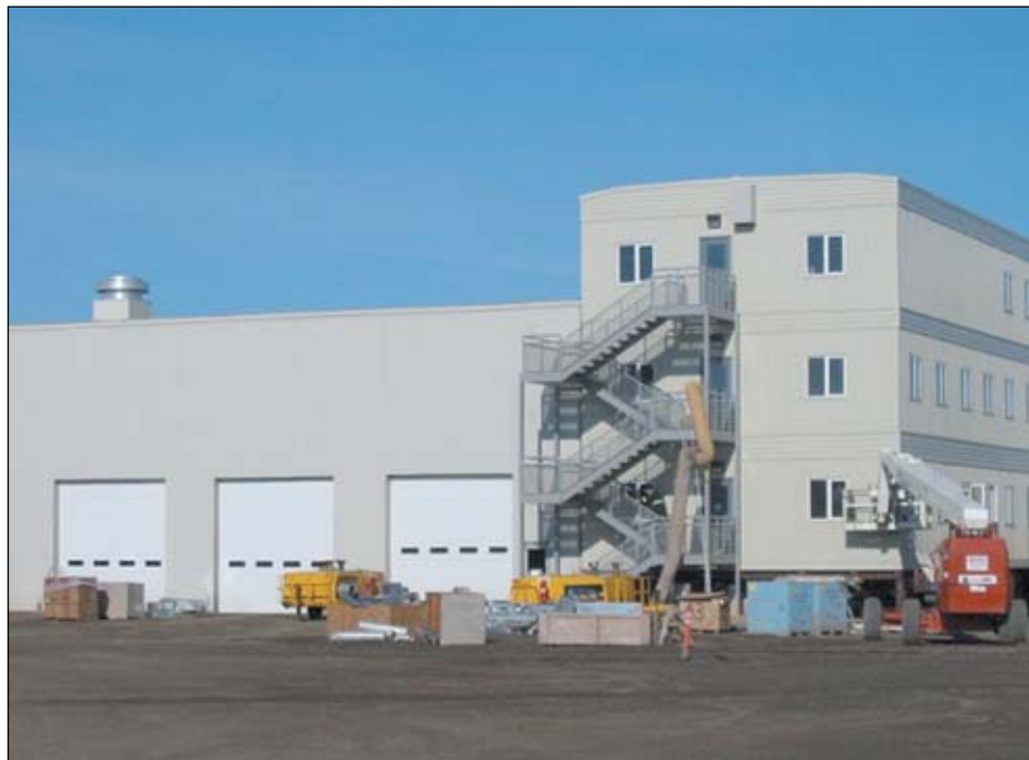
Travco modules built for Phillips Alaska's three-story emergency response center. The units were site installed by Nanuq Inc.
