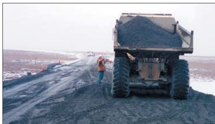
Placing gravel on the access road for the Tarn project at Kuparuk.
