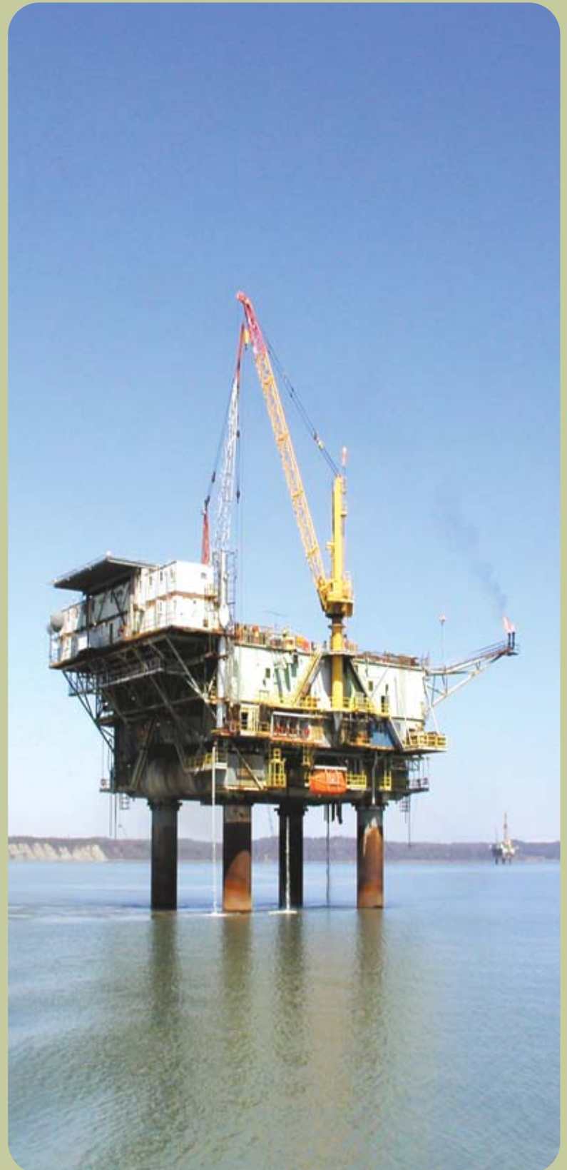
Cook Inlet Platform
