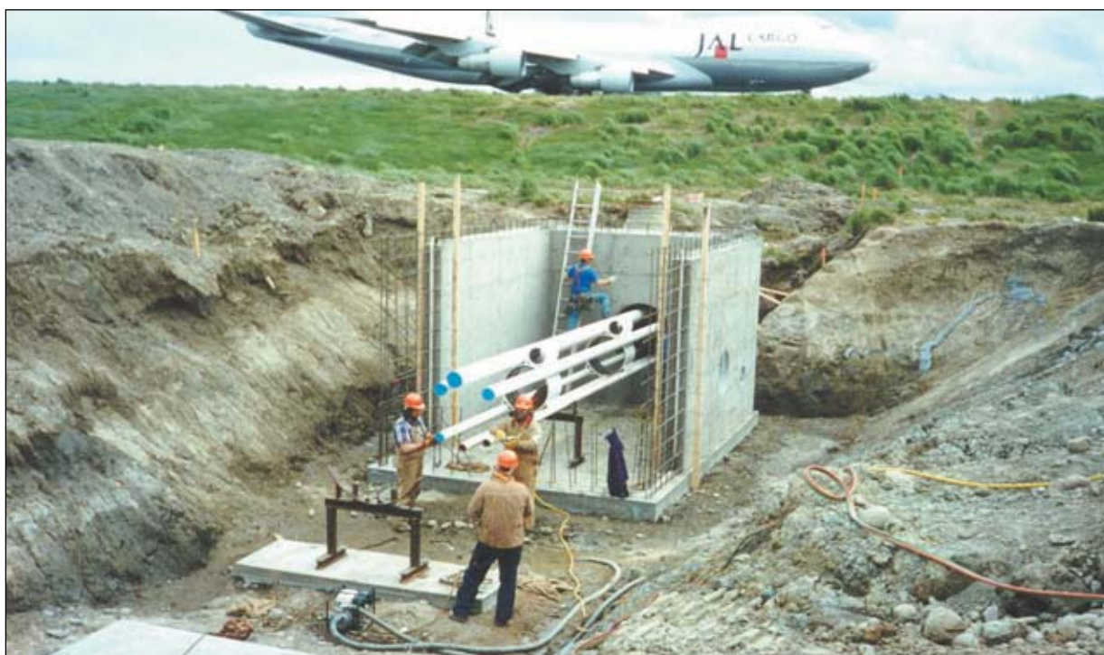
Sliding pipelines under the main runway at Ted Stevens Anchorage International Airport as part of a major upgrade to the fueling system at the airport
