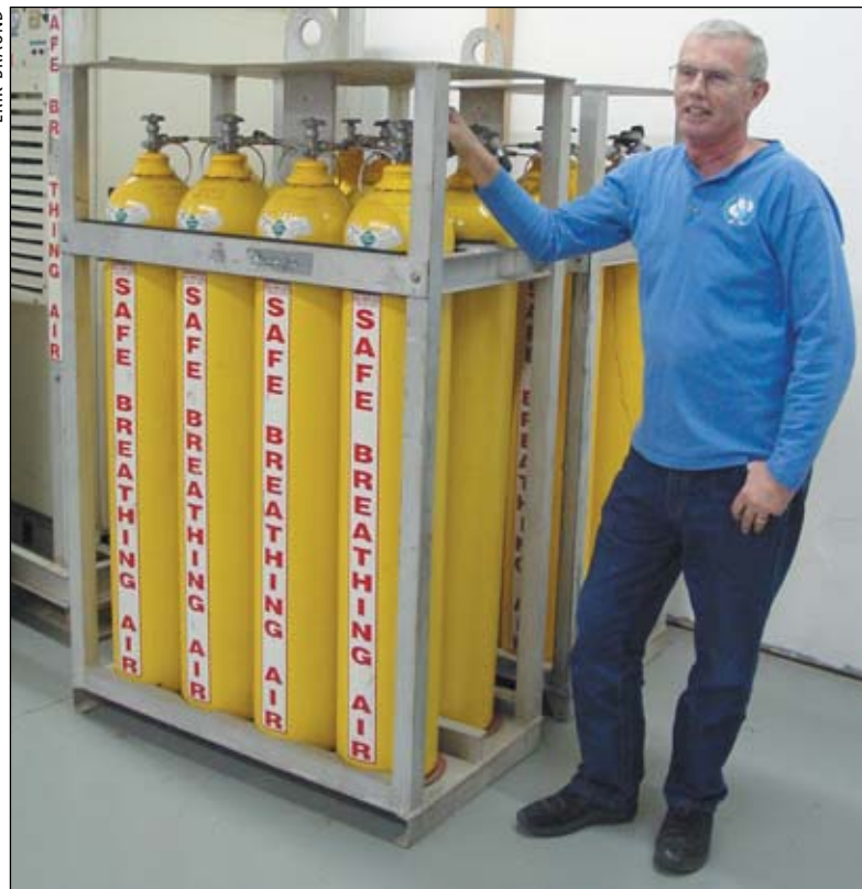
Well Safe’s Bob Pettit explains the breathing air cascade system to a customer. Cylinders are cascaded, or attached in a series, to each other and airlines are routed to manifolds or breathing air stations located around the rig where one or more individuals can hook up to the breathing air for long periods of time.
