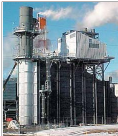
Great Northern Engineering participated in the design of this 40 megawatt gas turbine generator at Nikiski for supplying electricity to the Kenai Peninsula power grid. Exhaust gas from the turbine generates steam for use in nearby industrial chemical plants.
