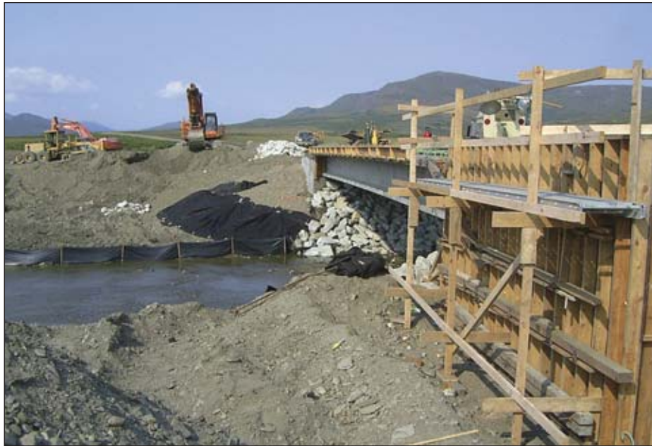
This summer's construction work on the Glacier Creek bypass road for NovaGold's Rock Creek mine near Nome.
