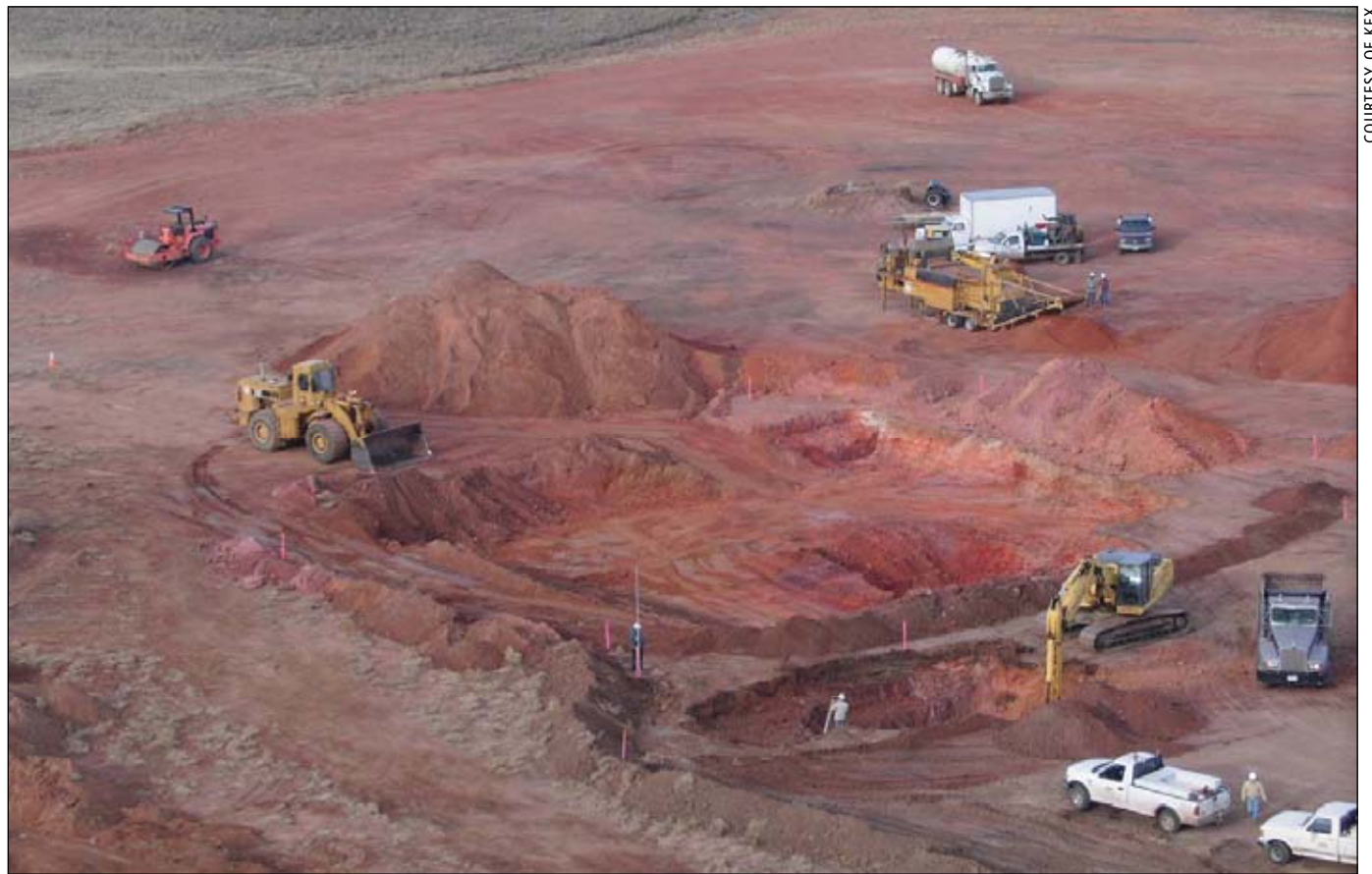
KFx is building a coal processing plant in Gillette, Wyo.
