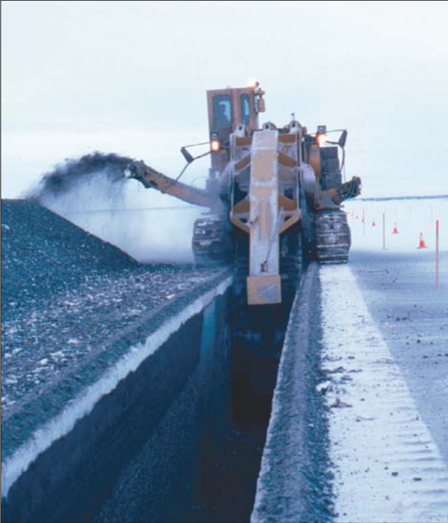
Trenching work near Deadhorse and Fairbanks in the winter of 2001-02 sought to verify the accuracy of North Slope gas producers' trenching estimates for the proposed gas pipeline from the North Slope to Lower 48 markets.
