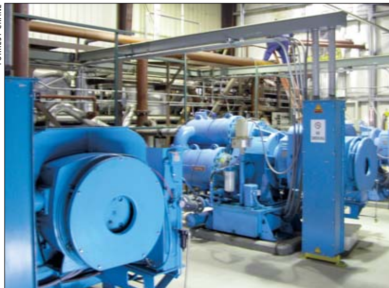
Air Liquide has an upgraded, FDA-approved, 35-ton-per-day air plant to supply the state with oxygen and nitrogen.
