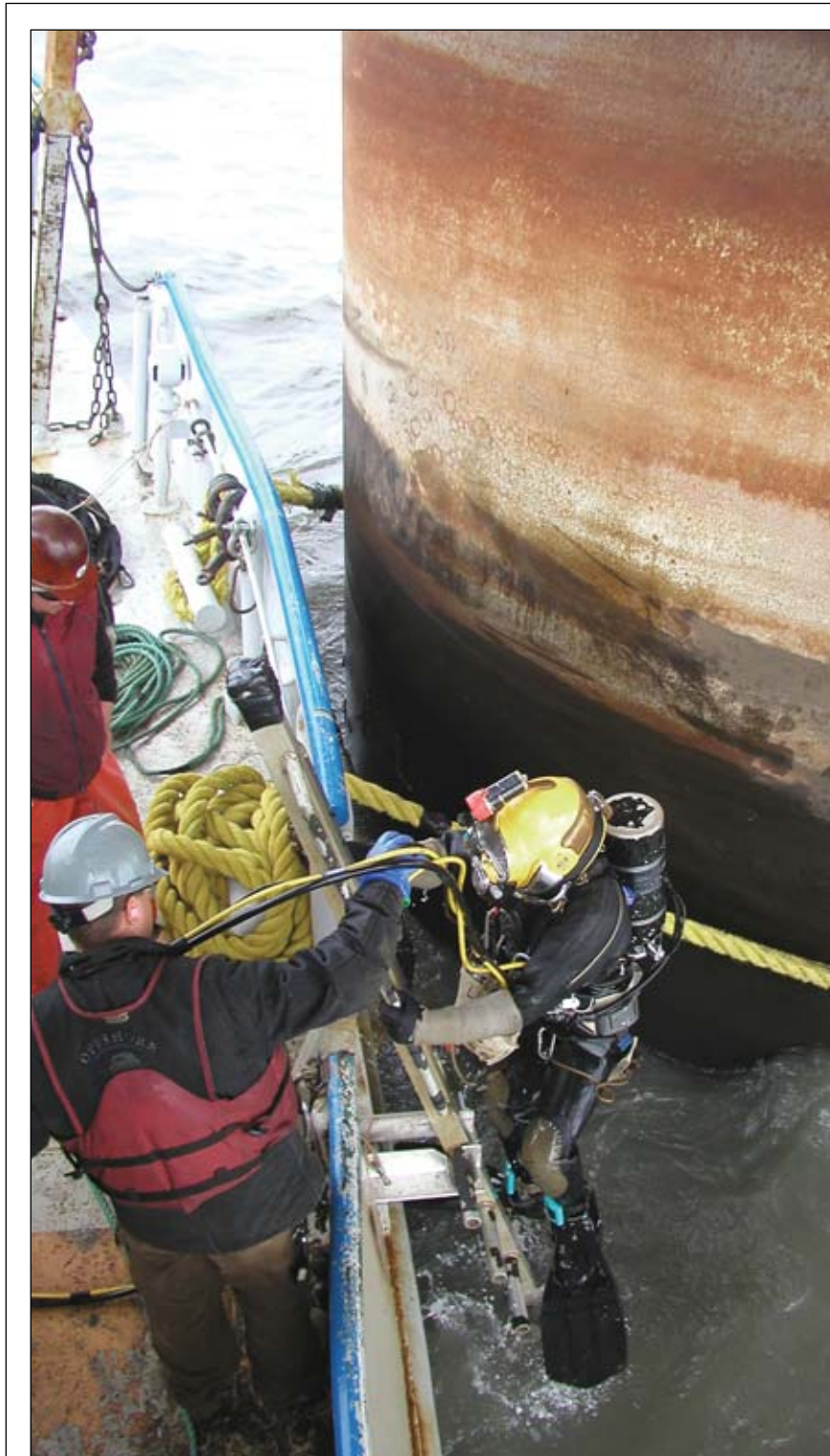
An Offshore Divers employee surfaces after working on a Cook Inlet platform.
