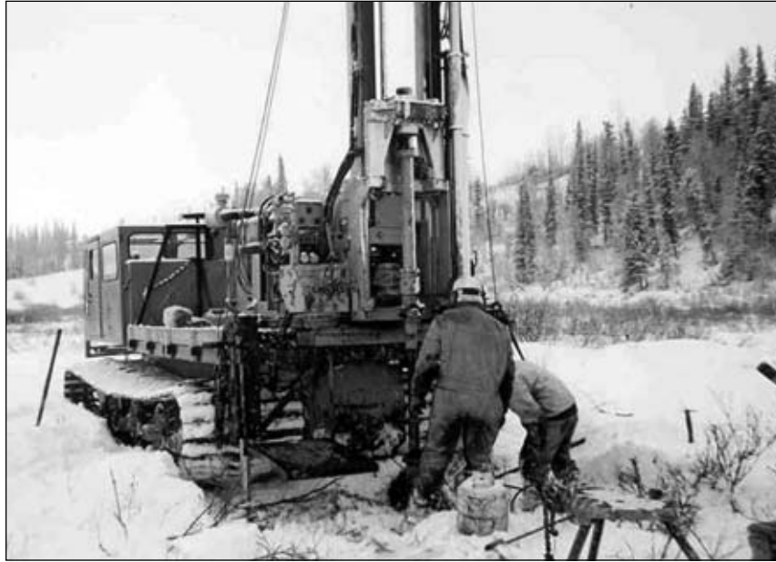
Michael Baker Jr. employees work on the Kenai-Kachemak pipeline corridor on Alaska's Kenai Peninsula.
