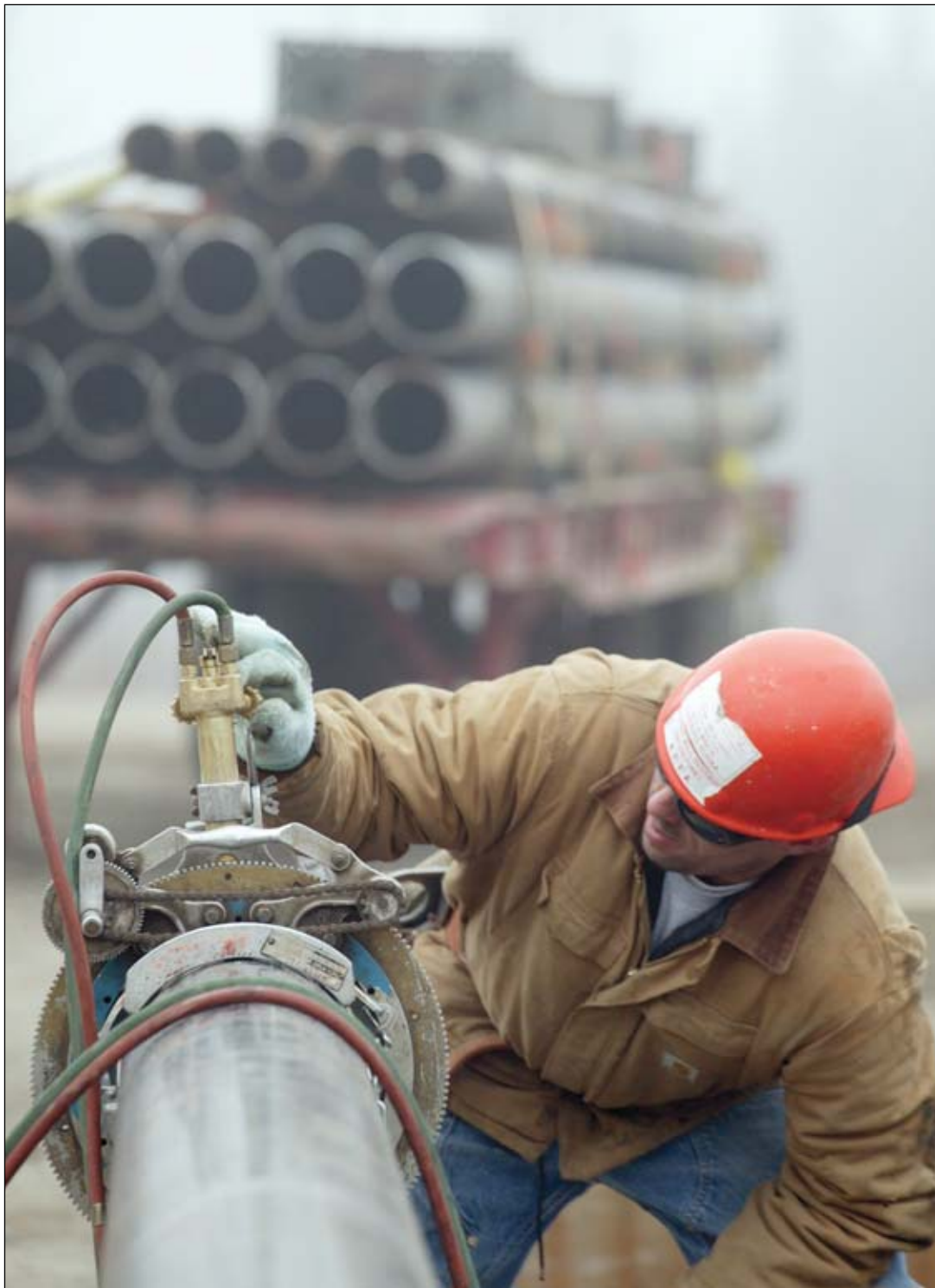
A worker cuts drill pipe in this image captured by industry photographer Judy Patrick.
