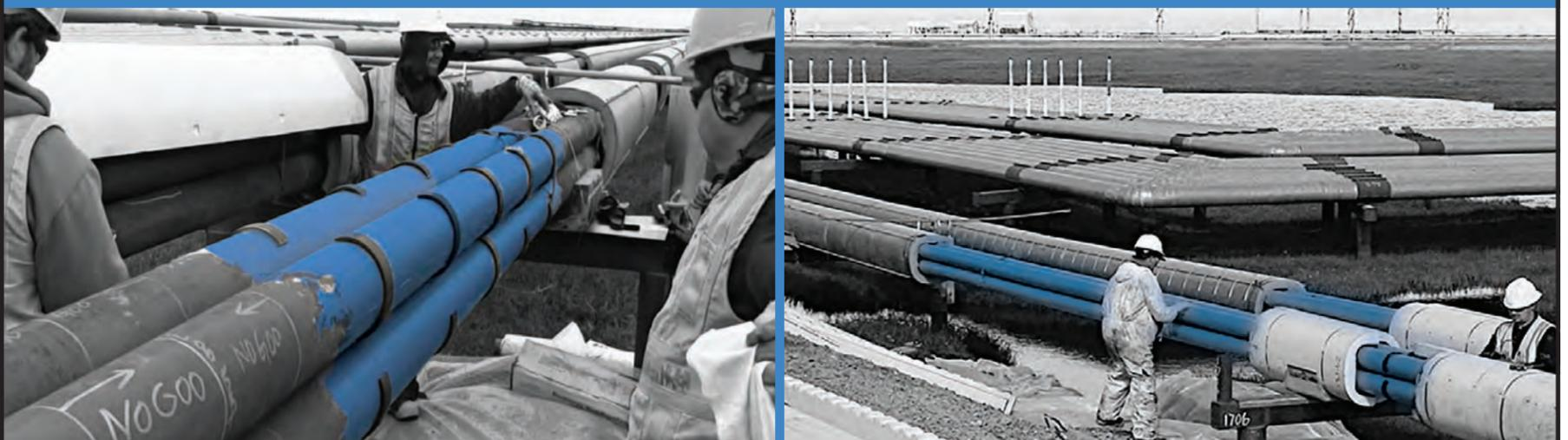
Polyguard Products has introduced a really different type of corrosion protection to address Alaska’s corrosion problems. ReactiveGel® (nicknamed “BlueGoo®” by Oil Patch users) is a patented product which reacts with steel surfaces to form a microscopically thin glasslike surface. This glasslike surface will not corrode.
