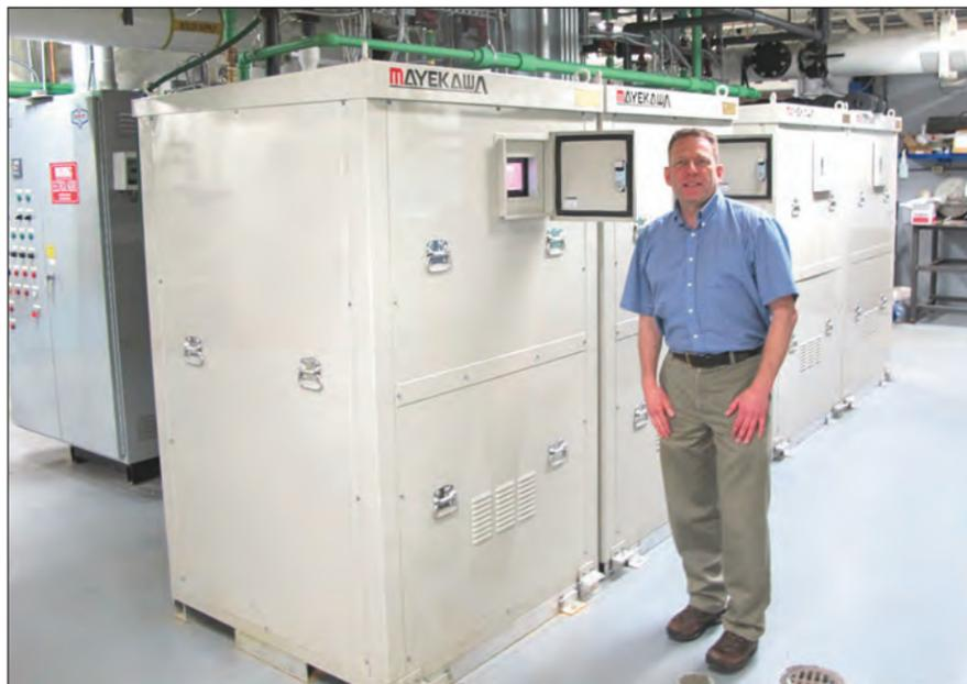
Darryl Schaefermeyer, special projects director for the Alaska SeaLife Center, in front of a bank of four state-of-the-art heat pumps that use carbon dioxide as refrigerant and provide heat for the center.
