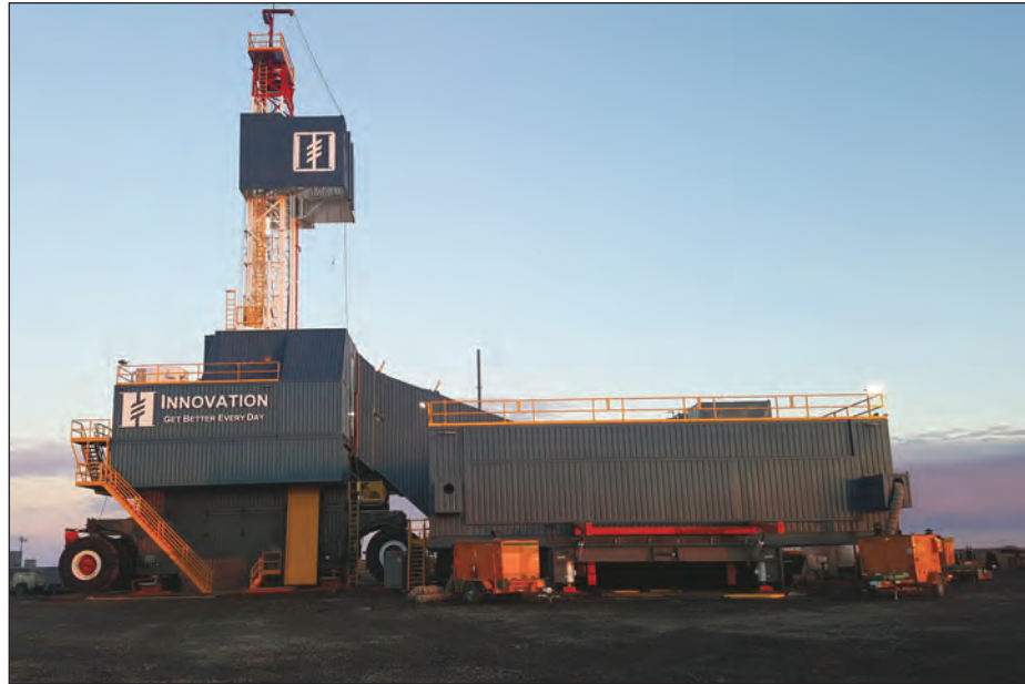
The new Innovation drilling rig which Hilcorp Alaska had built for use on the North Slope is very mobile and can access wells on 10-foot spacing.
