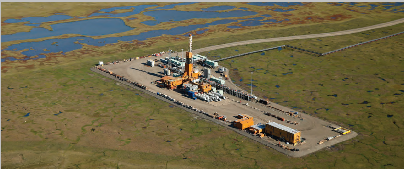
Doyon Rig 19 on ConocoPhillips' CD-3 drill site in the Colville River unit
