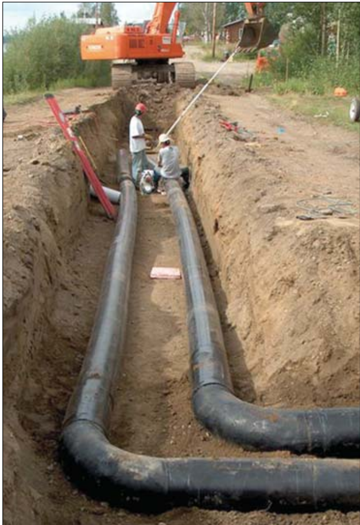
MWH designed and oversaw the installation of nearly 30,000 feet of water and sewer mains for the community of Tanana.
