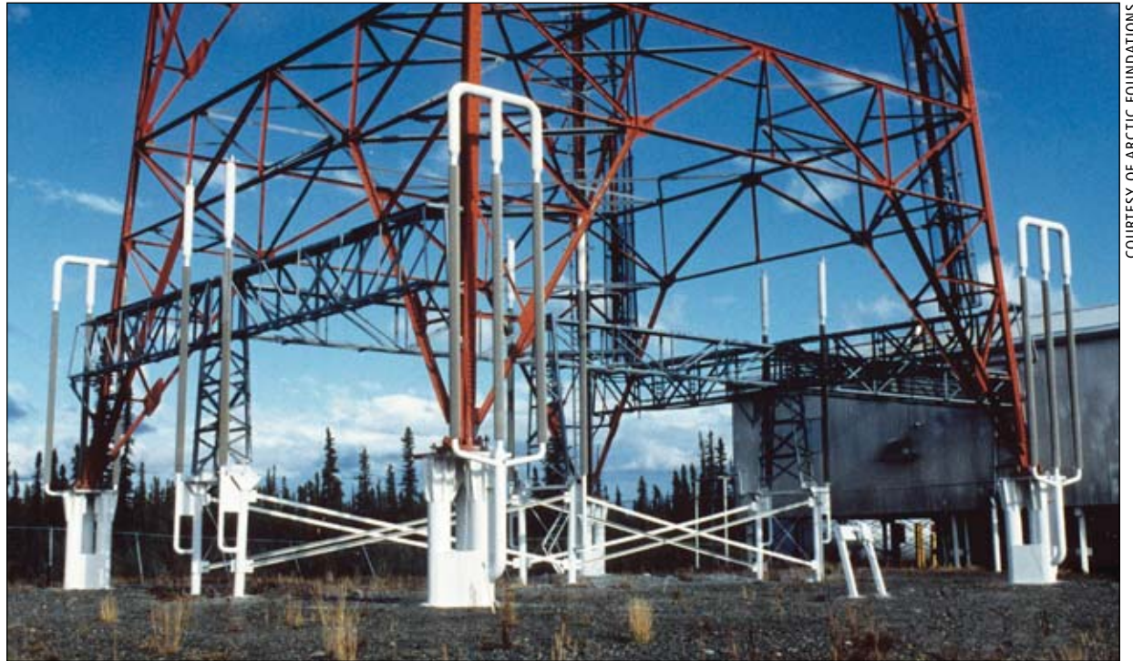
At the Aurora communications tower, Thermosyphon units installed by the Corps of Engineers in 1960 are still functioning and maintaining their permafrost stability today. Erv Long, owner of Arctic Foundations developed the Thermopile system and patented his thermal transfer process in the late 1950s.
