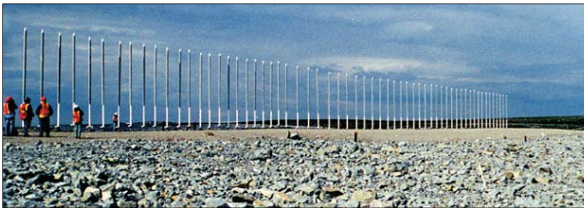
Above, Arctic Foundation's hybrid Thermosyphon Technology is a well-established technology ideally suited to containment and dams. A frozen dam can be even more effective than a traditional type because freezing can more effectively seal multiple soils types in and below the dam as evidenced at the Panda Dam in Northwest Territory Canada. At right, Usibelli Coal Mine: a view from Two Bull Ridge looking at the land reclamation on Poker Flats Mine
