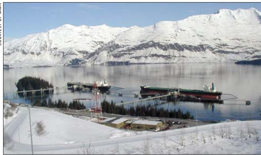
MWH designed improvements to the Ballast Water Treatment facility as well as water supply and domestic wastewater at the Valdez Marine Terminal.
