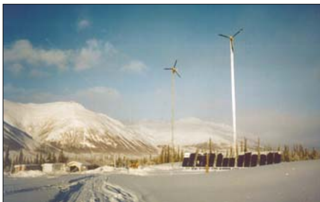
For the FAA Chandalar Lake radio navigation beacon, MWH designed and installed an innovative multi-fuel power system that utilizes an array of solar panels, wind turbines, and diesel generators dramatically reducing fuel consumption.
