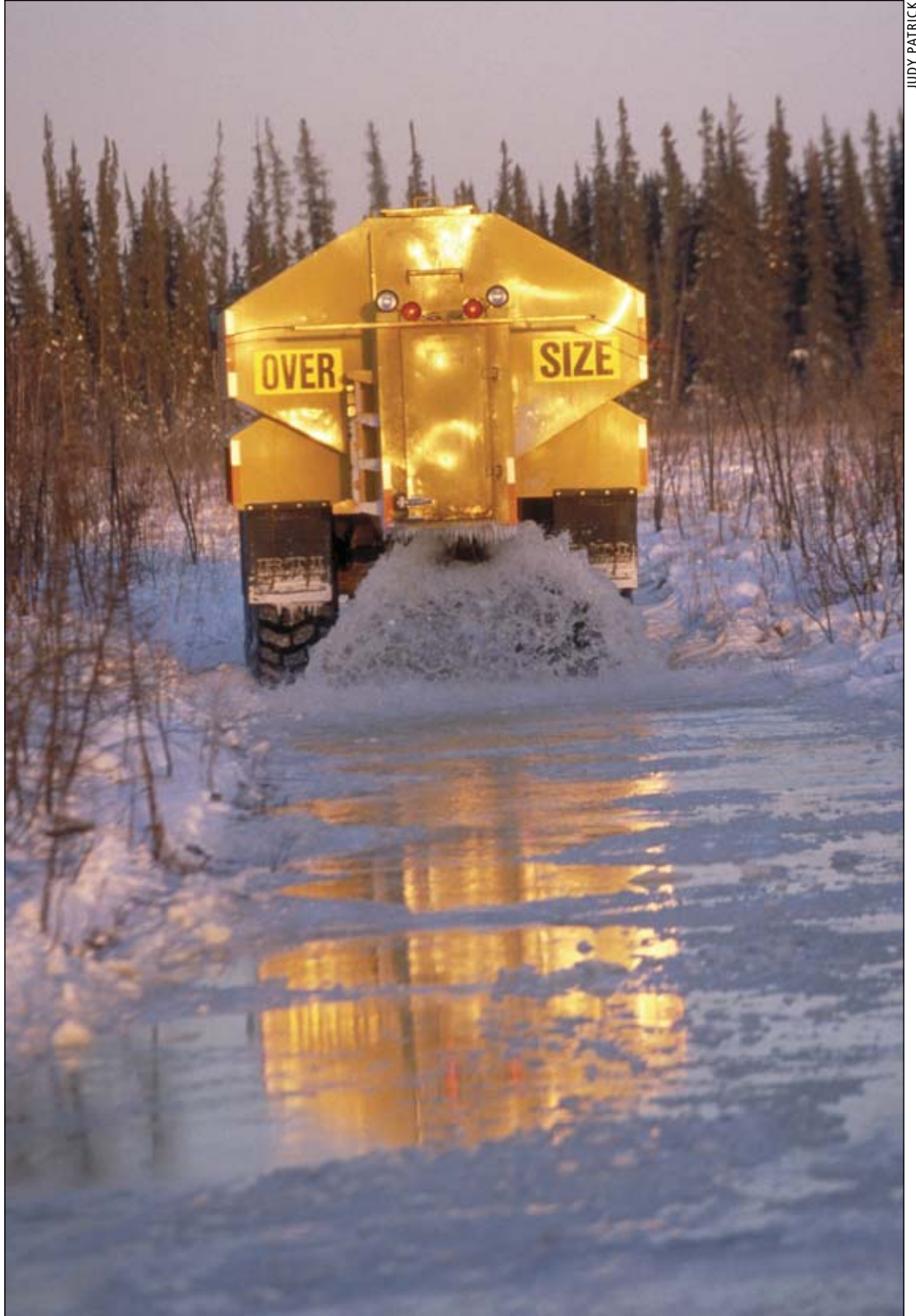
A Cruz Construction water truck works on the construction of an ice road. The company specializes in winter ice roads, ice pads, land clearing and pioneer roads, exploratory support, off-highway transport, remote fuel transportation, and heavy civil construction.
