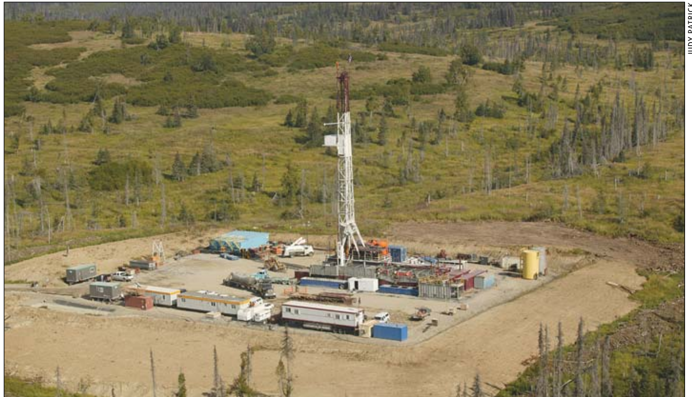
Aerial photo of Nabors Alaska rig 129 on the Red Pad in Unocal's Nikolaevsk exploration unit on Alaska's southern Kenai Peninsula. The photo was taken on Aug. 13. Unocal has drilled and is evaluating two exploration gas wells at Nikolaevsk, the Red No. 1 and the Red No. 2. (See story in last week's Petroleum News.)
