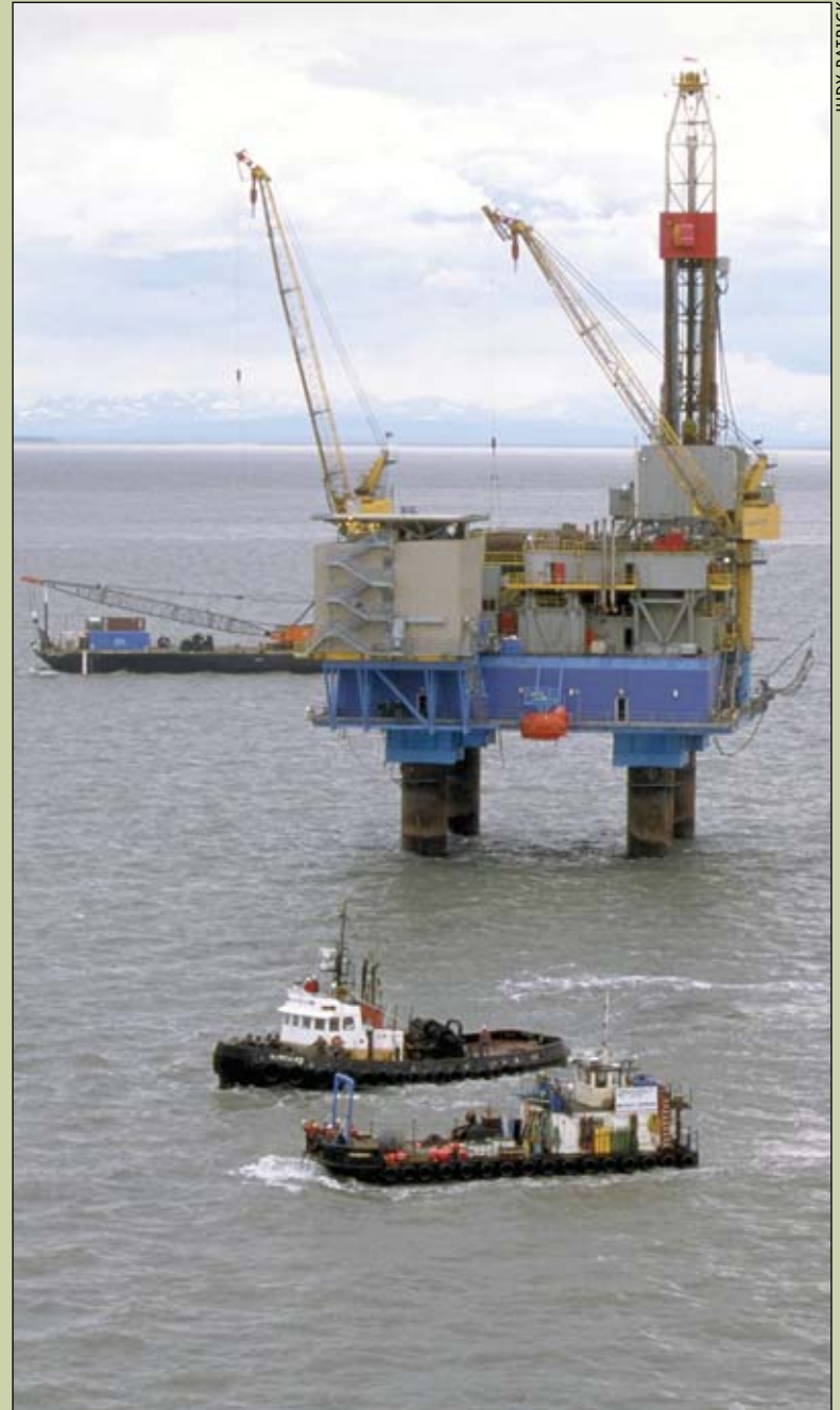
The Osprey platform during the pipeline installation phase. Crowley Alaska's tugboat, Sea Breeze, and American Marine Corporation's vessel, Shamrock, both were instrumental in the pipe pulling operation.
