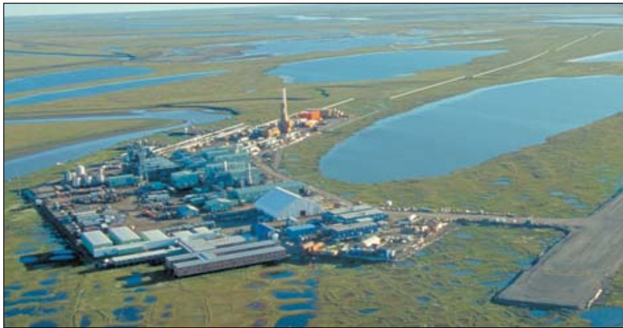
The Alpine field on Alaska's North Slope
