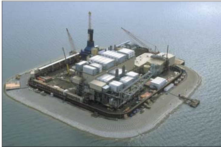
The Northstar unit straddles state and federal waters in the Beaufort Sea, with the five-acre production island rising out of a depth of about 39 feet. The island is heavily fortified against sea ice.
