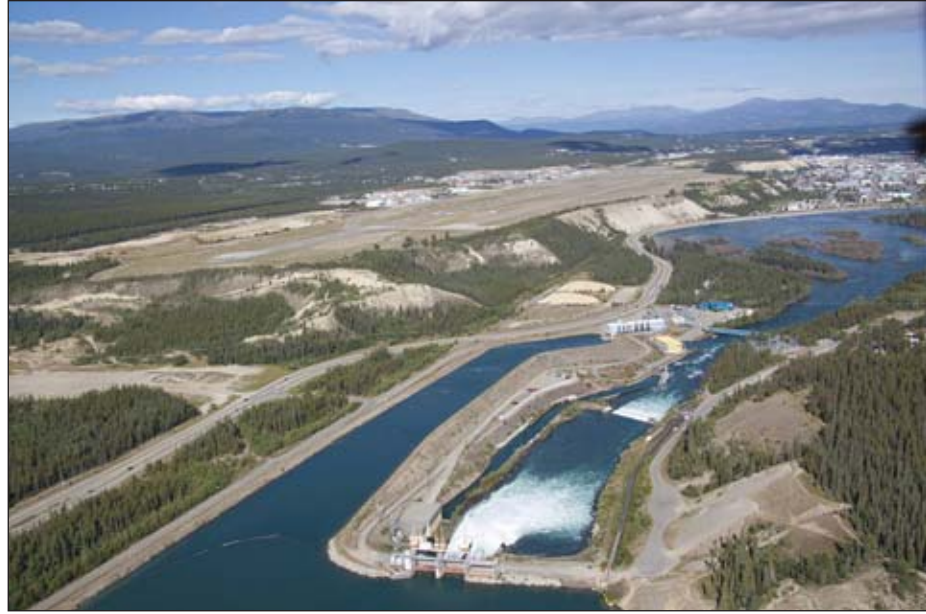
The Whitehorse dam, foreground, on the Yukon River is the Yukon Territory's biggest energy source, with four hydro generators and seven diesel generators. Whitehorse downtown is in the upper right and the airport is in the photo's center.
