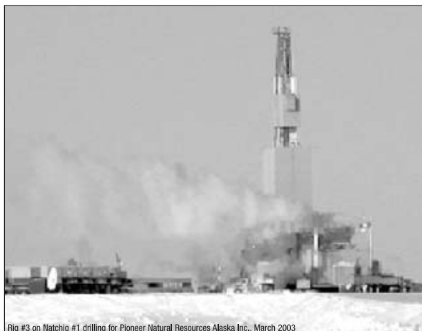
Rig #3 on Natchig #1 drilling for Pioneer Natural Resources Alaska Inc., March 2003
