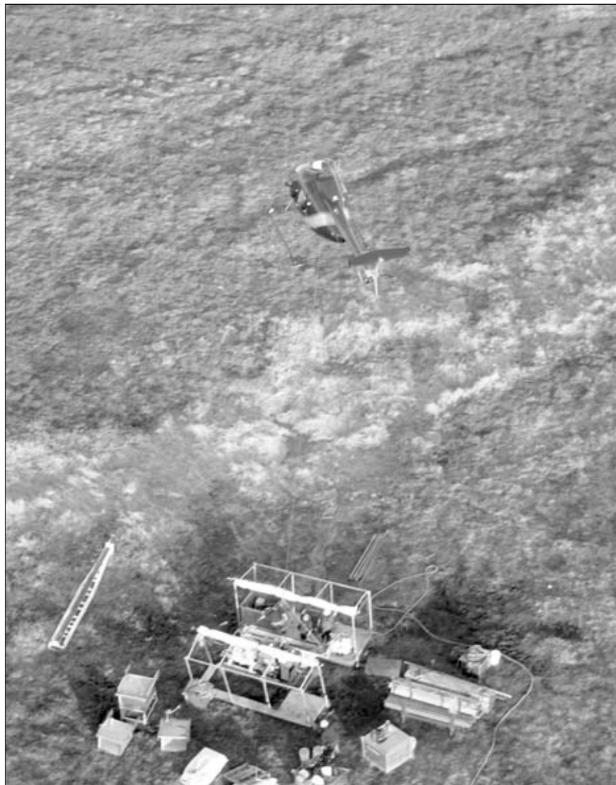
Due to the difficult superlative challenges, helicopters play a vital role in moving materials and manpower
