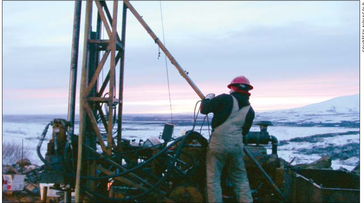
Drilling site at NovaGold's Rock Creek
