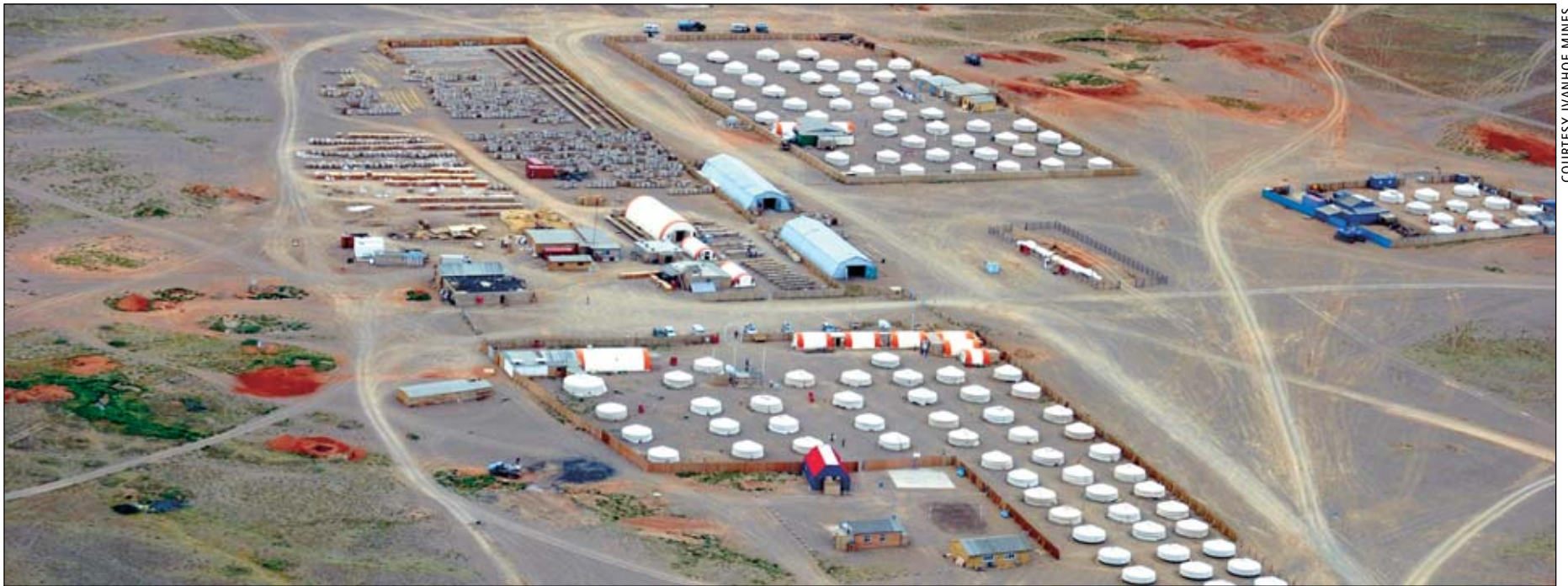
Aerial view of Ivanhoe's Mongolian Oyu Tolgi copper-gold facilities
