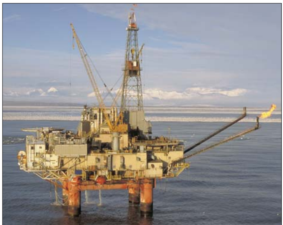
Unocal's King Salmon platform in Cook Inlet
