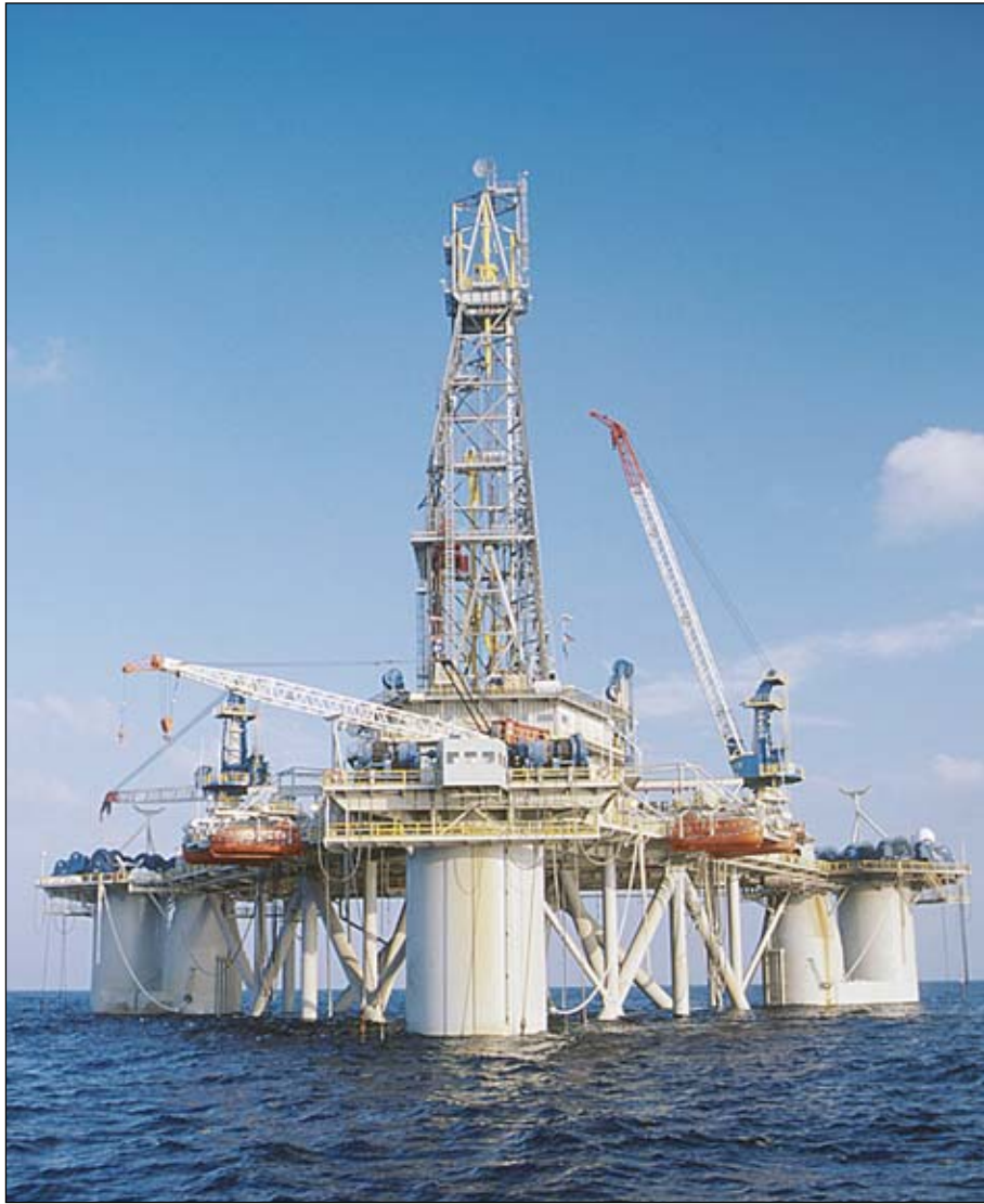
Amos Runner drilling rig
