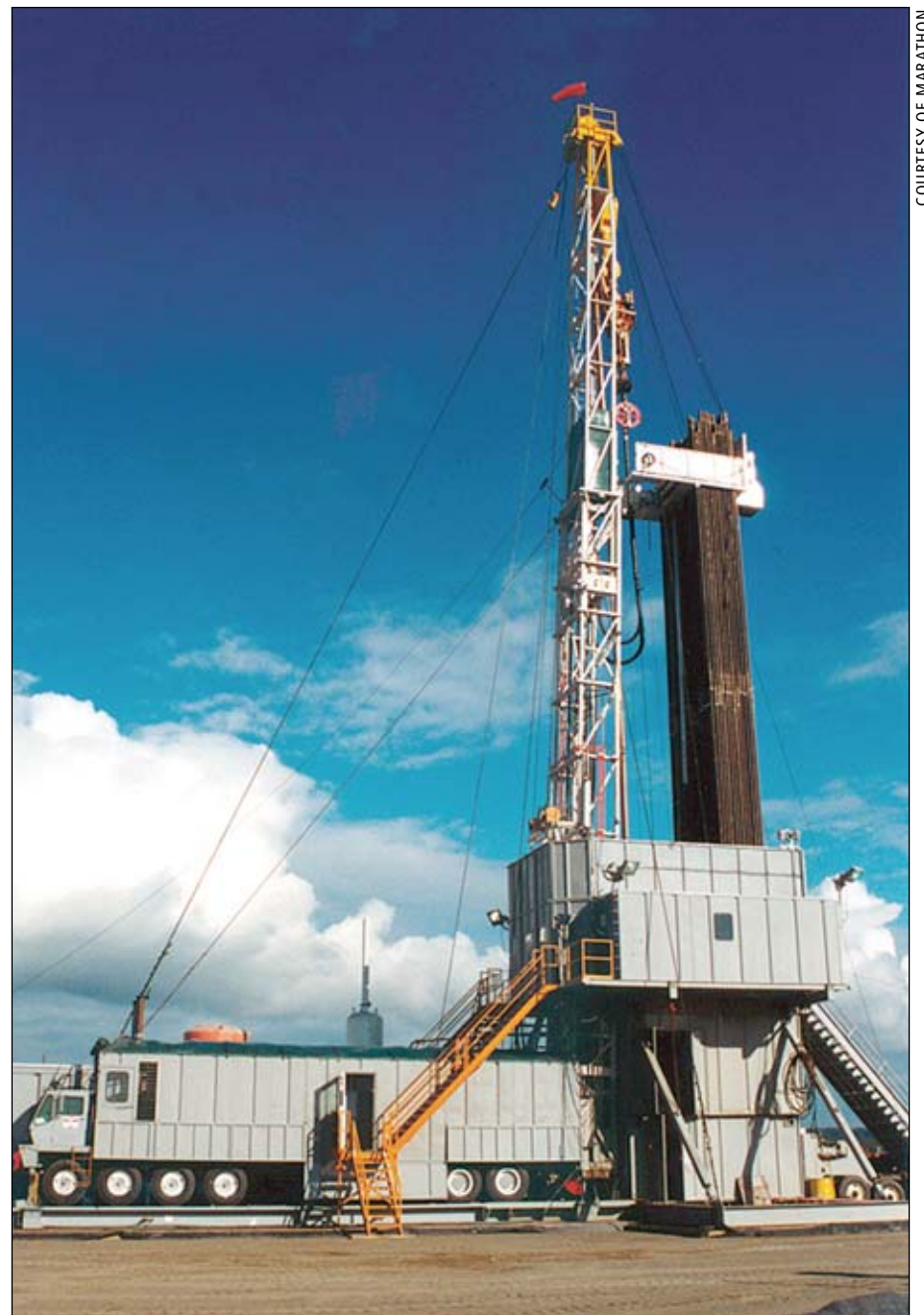
Marathon commissioned the Glacier drilling rig during 2000. The rig was specially designed to meet Marathon's Cook Inlet needs, minimizing cost and environmental impacts. The Glacier rig has drilled more than 27 wells and 250,000 feet of hole since commissioning.
