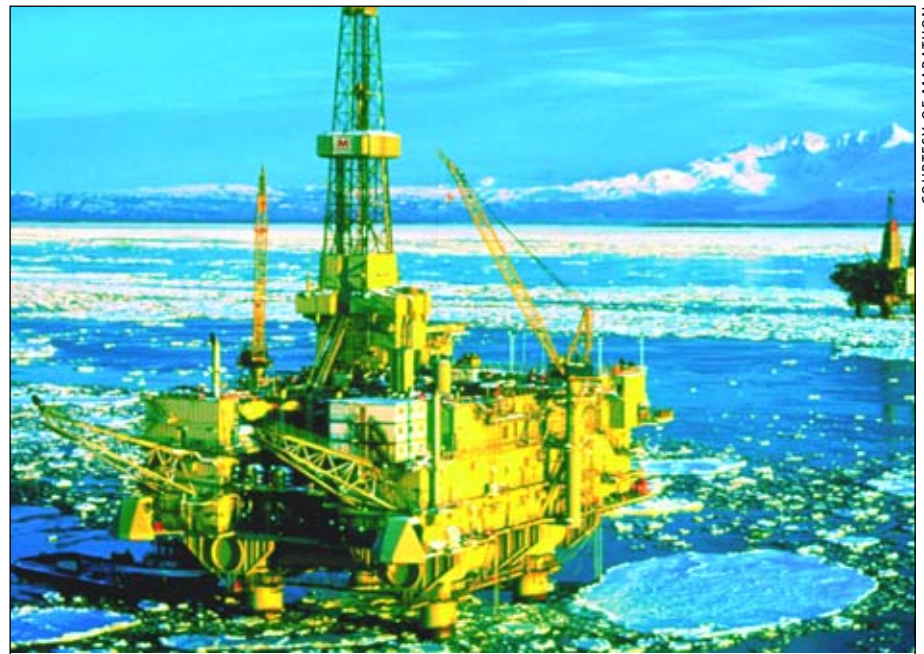
Marathon installed the Steelhead platform, the largest offshore platform in Cook Inlet, in 1986.
