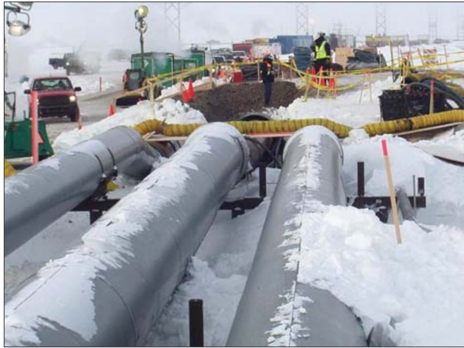
Cleaning up the oil spill in the caribou crossing in the Gathering Center 2 transit line at Prudhoe Bay
