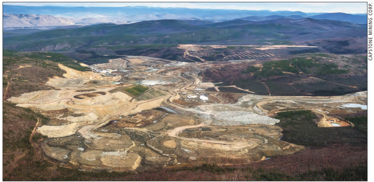
Going into 2016, Capstone Mining reported plans to temporarily halt operations at its Minto copper-gold mine in 2017. With mining now advancing at the high-grade Minto North pit, the company is anticipating significantly higher copper production at this Yukon Territory operation in the second half of 2016.
