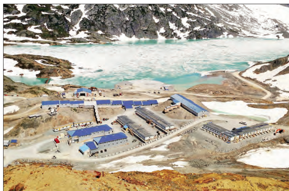
Since this photo was taken, about a year ago, Pretium Resources has made significant progress on development at its high-grade Brucejack gold mine project in northwestern British Columbia. With the mill building now nearly enclosed, the company remains on schedule to begin commissioning the underground mine in mid-2017.
