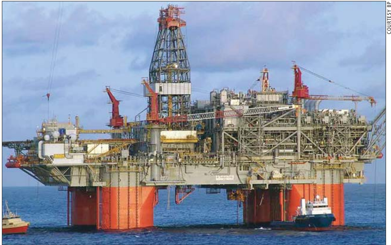
At 50,000 tons, Thunder Horse is among the largest production drilling semi-submersible platforms in the world.
