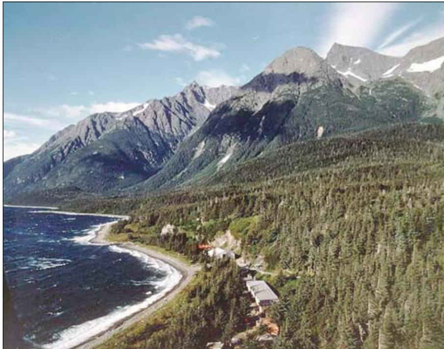
The camp at the Kensington gold project being developed by Coeur d'Alene Mines Corp. some 45 miles north of Juneau, Alaska.
