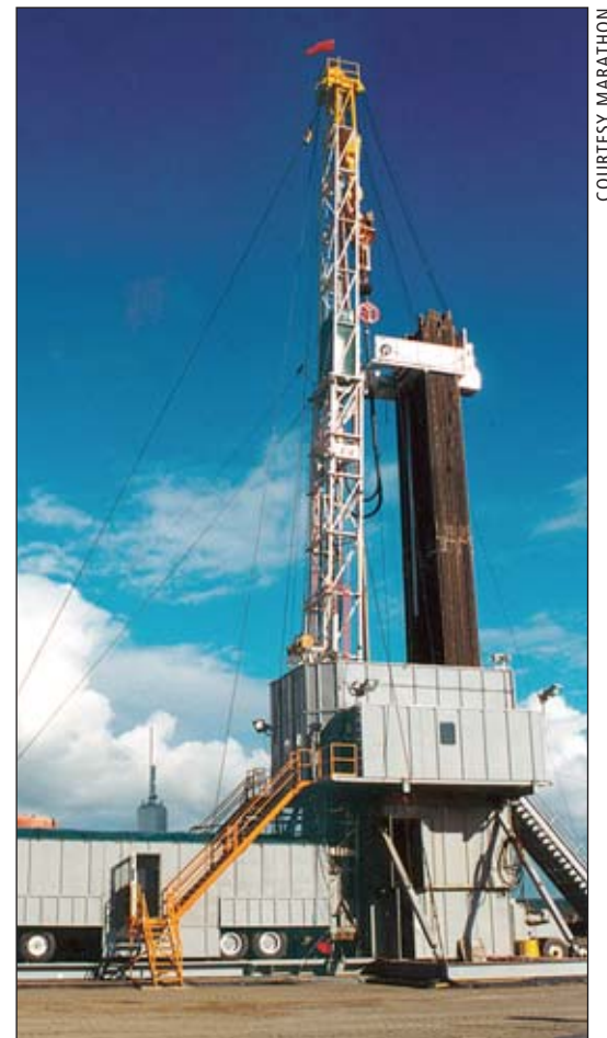
Marathon Oil Co.'s Glacier No. 1 drilling rig. Will it be heading to the North Fork unit in the southern Kenai Peninsula to drill for oil for Armstrong Cook Inlet?
