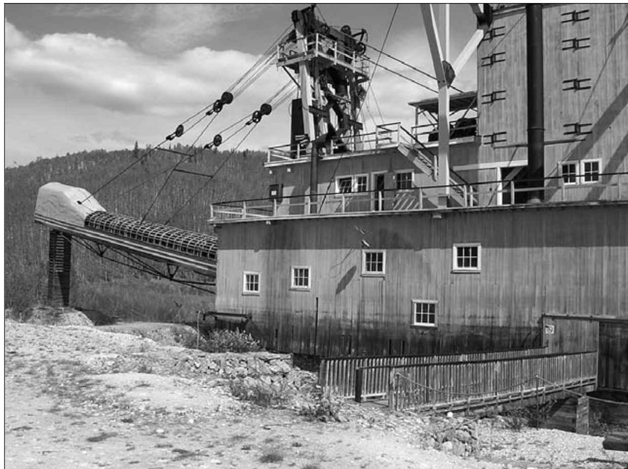
Dredge No.4, assembled in 1913, is now a tourist attraction at the location where it used to work, a few miles outside Dawson City
