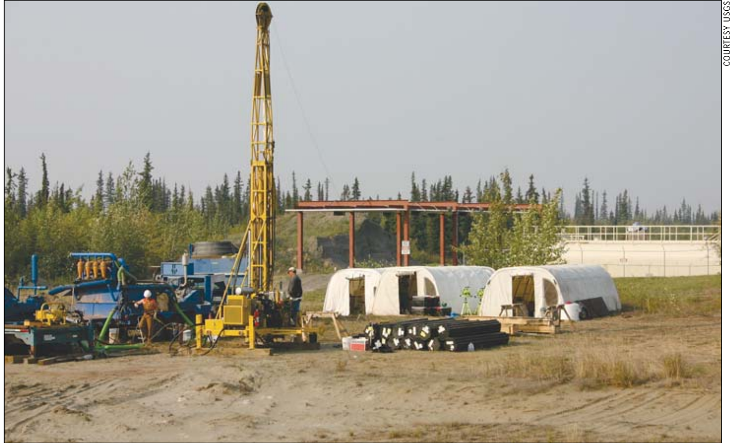
The lightweight CS 1000 drilling rig in operation at Fort Yukon.
