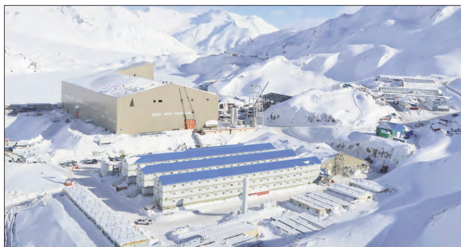
At the end of March, Pretium Resources was finishing construction at the Brucejack gold mine project. With power now delivered to site, the company plans to begin processing ore by mid-April.
