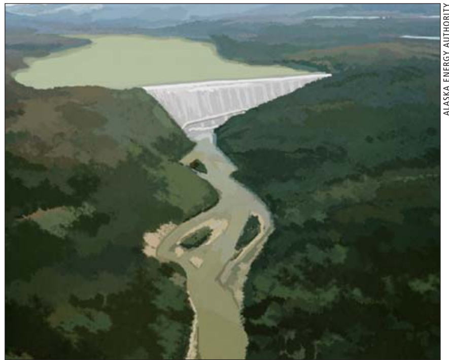
The proposed Watana Dam would stand about 700 feet high and create a reservoir 39 miles in length.
