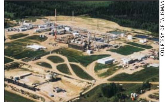
Talisman Energy has begun construction of a 10-megawatt co-generation power plant at its Edson natural gas processing facility, the Calgary-based company said June 21.
