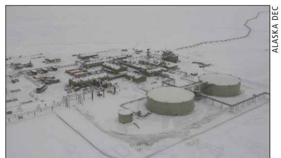
Pump Station 1 and the storage tanks used to hold oil field production while the trans-Alaska pipeline is shut down.
