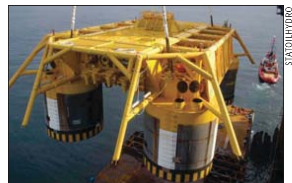
A subsea template being lowered into the sea at the Ormen Lange field.
