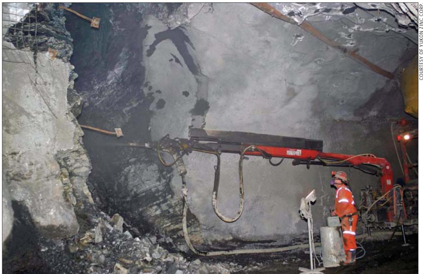
A mine worker uses a “shotcreting” machine to spray a concrete material onto vertical and overhead surfaces of the underground workings at the Wolverine Project in Yukon Territory in preparation for the start of production in mid-2010.
