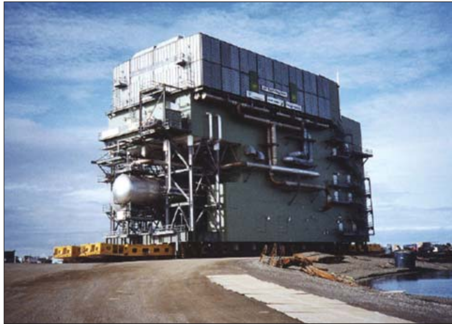
Operators at Prudhoe Bay launched oil production with relatively modest waterflood and gas injection capabilities. This compressor plant was a part of the original development.
